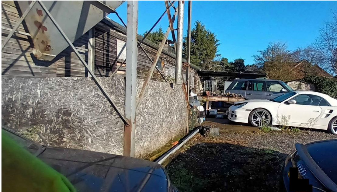
View looking northeast, with the disused silo and building C in the left foreground of the photograph
