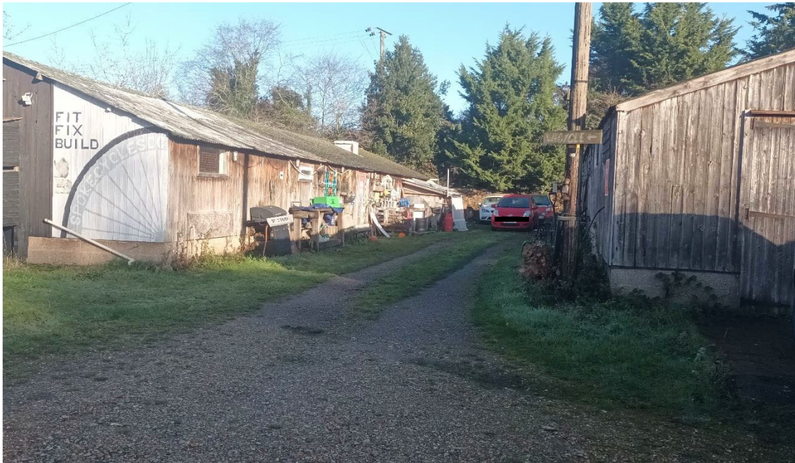
View looking north, northeast, between the existing structures used for vehicle maintenance.
