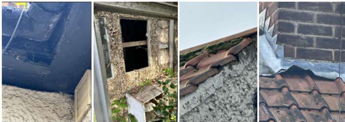
Figure 4 Potential bat roost locations on site.
