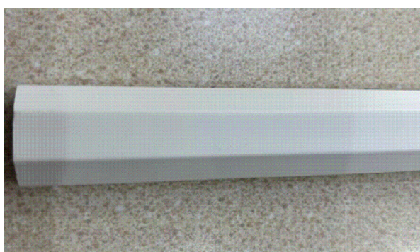
PROPOSED CHAMFERED GLAZING BAR PROFILE TO MATCH EXISTING WITH INTERNAL OVOLO PROFILE
