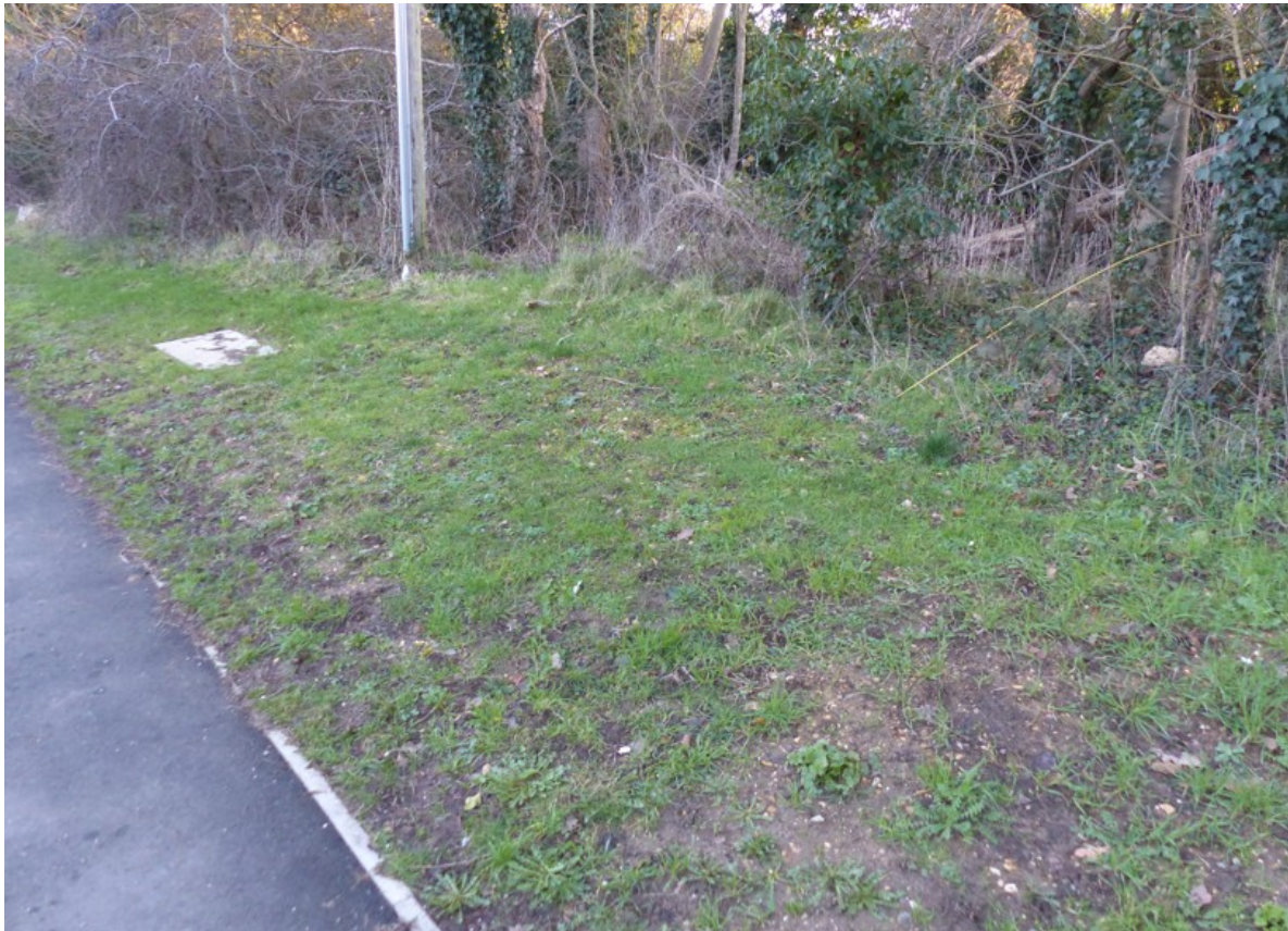
Fig. 3 The differences in levels between the highway and the wood mean that cellular confinement product is impractical here
