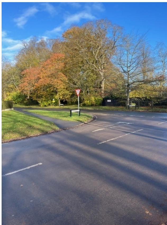
Figure 5.6 – Pedestrian crossing point over Church Lane, dropped kerbs present (looking northeast)
