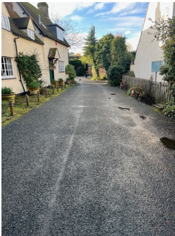
Figure 5.11 – Unnamed Road leading to Footpath 003, no footway provision present
