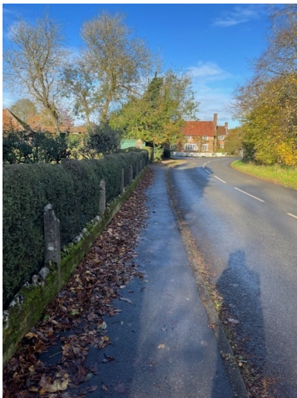
Figure 5.3 – Existing footway on the western side of School Lane, between Church Lane and Chequers Lane (looking north).
