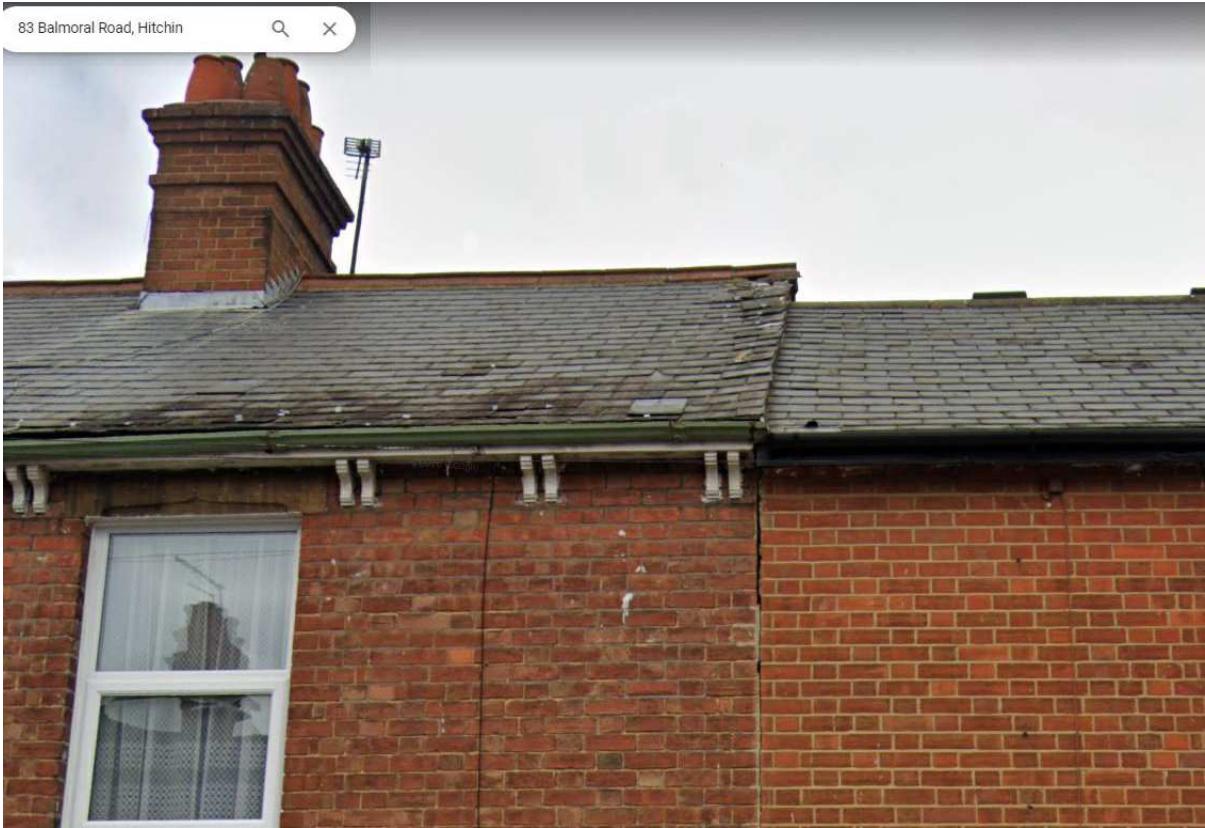
Boundary between 83 Balmoral Road (on the left) and 84 Balmoral Road (on the right)
