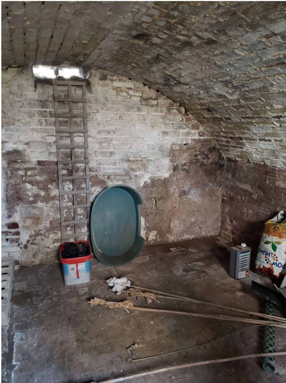
Cellar / Underneath Outbuilding
