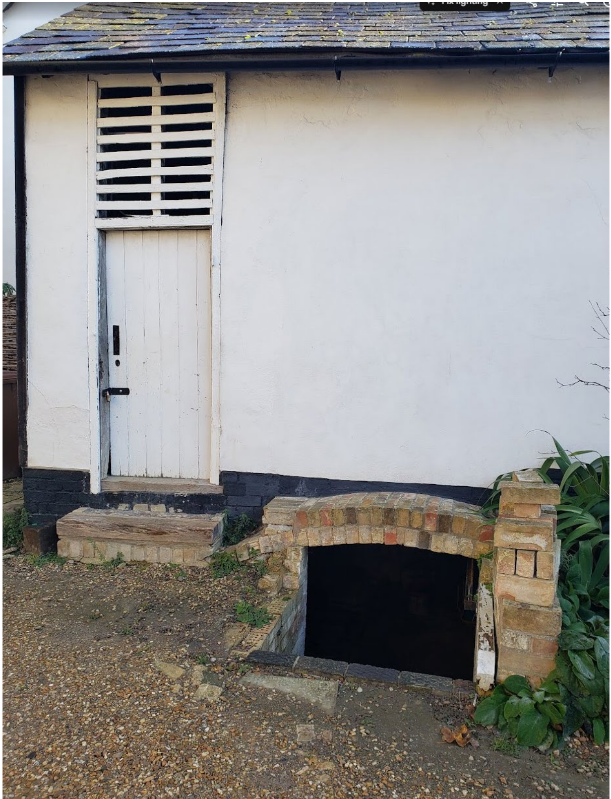
Outbuilding > Courtyard > Cellar Access
