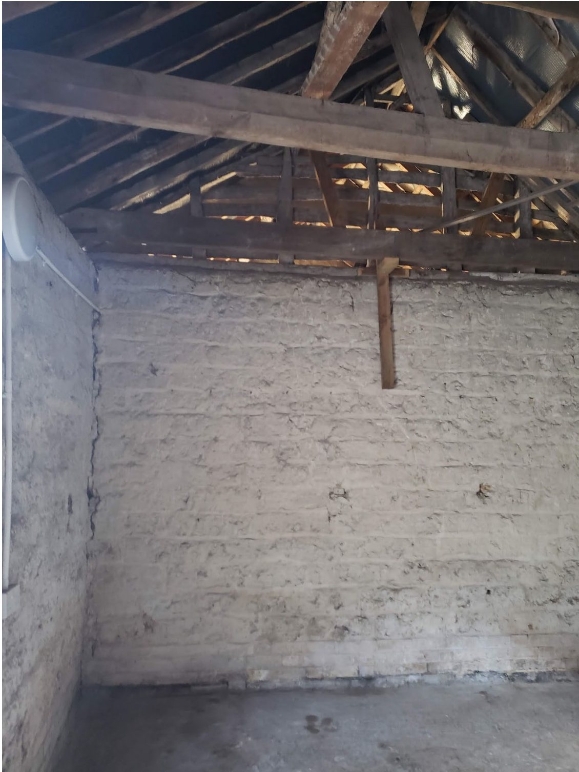
Clunch Wall > Central Wall / Outbuilding
