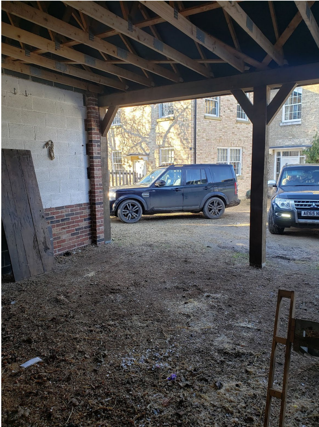
Existing Two Bay - Cart Lodge
