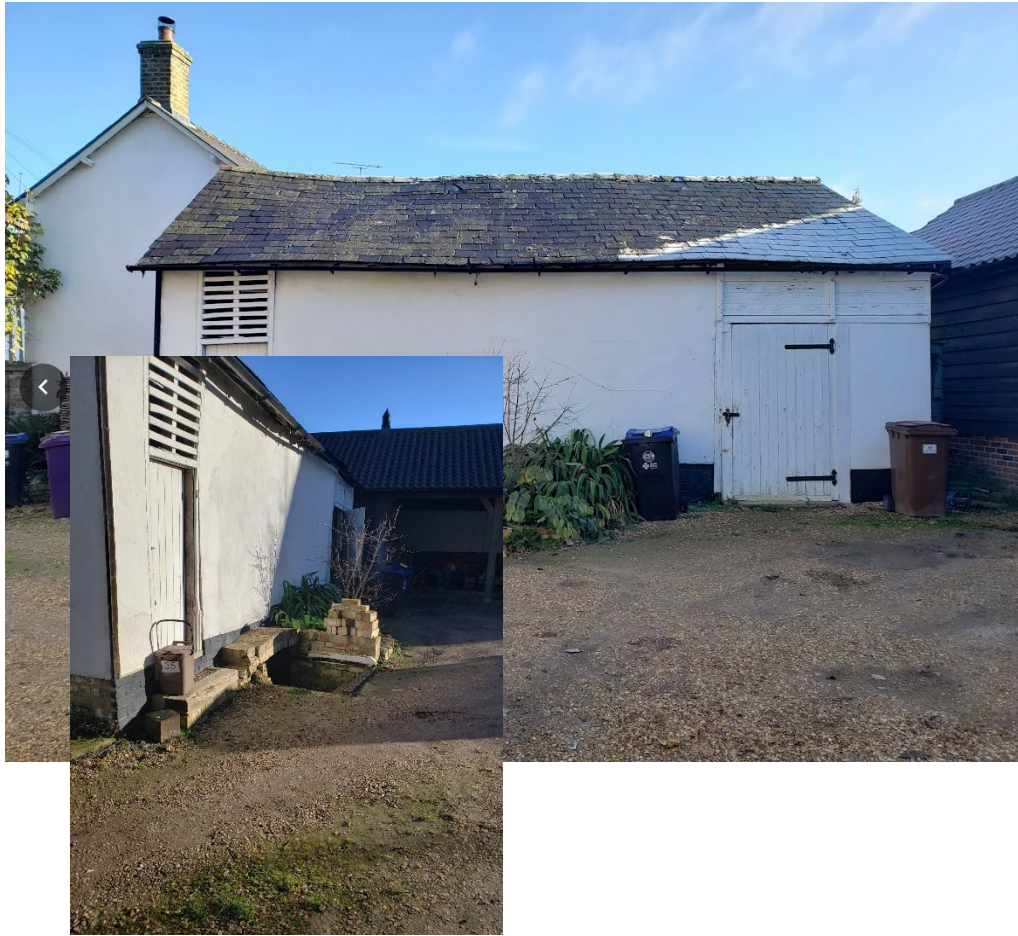
Outbuilding > Courtyard > Cellar Access
