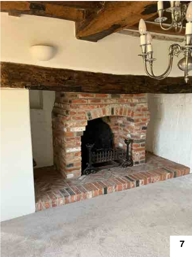
Interior - key views ground floor 1/2
