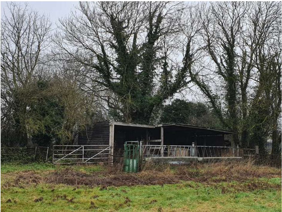
Existing agricultural building in north east site
