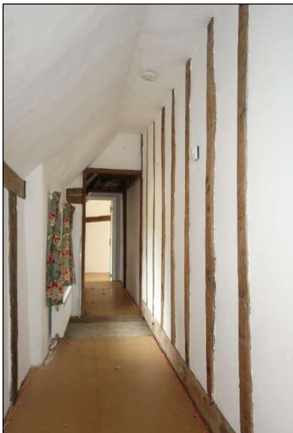
Plate 34: View looking E along first floor corridor showing exposed timber-framed panels
