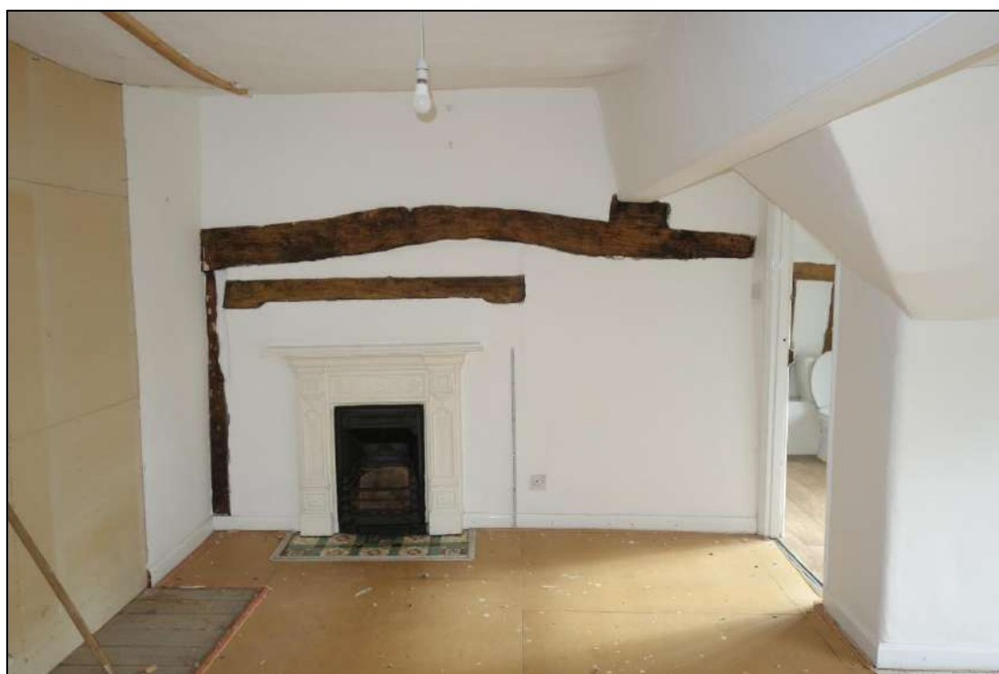
Plate 37: Internal view looking E showing E end of Bedroom 1 with smoke-blackened beam in wall, above 19 th century fireplace surround and grate
