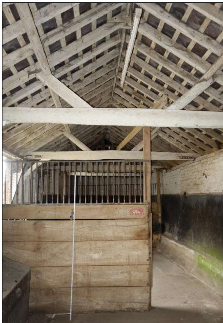
Plate 68: View looking S showing loose box partitions and open roof structure in S bay of weatherboarded stable range
