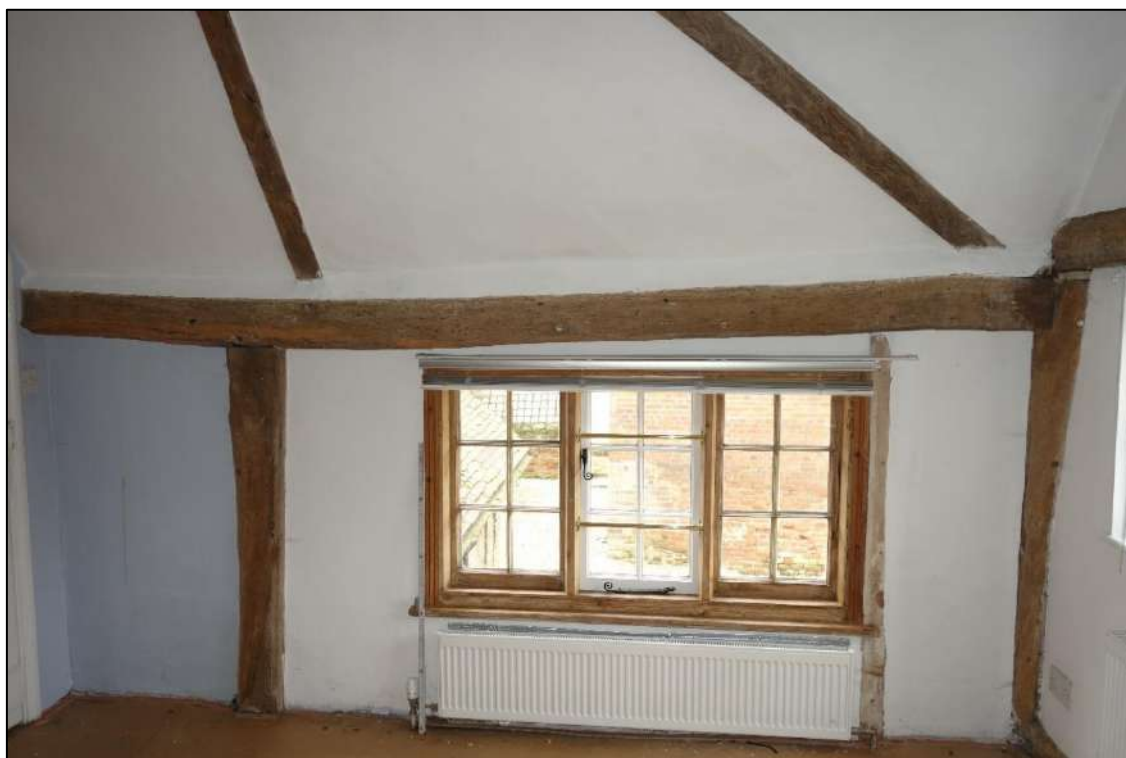
Plate 45: View looking W showing W wall of Bedroom 2 with mullioned window and exposed timber-framing
