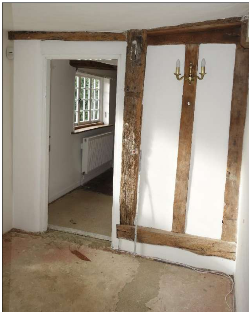
Plate 17: Internal view looking ESE showing lobby between sitting room and living room with close-studded timber framing
