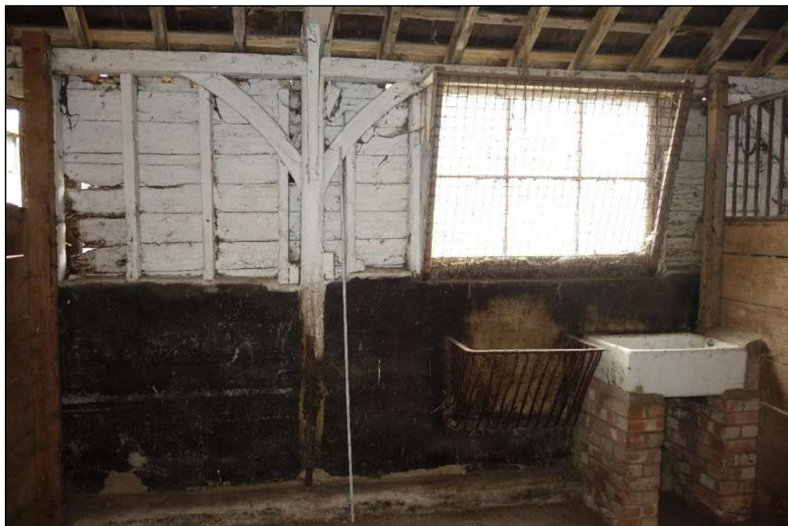
Plate 70: View looking E showing vertical wall posts and studding along E wall of stable range
