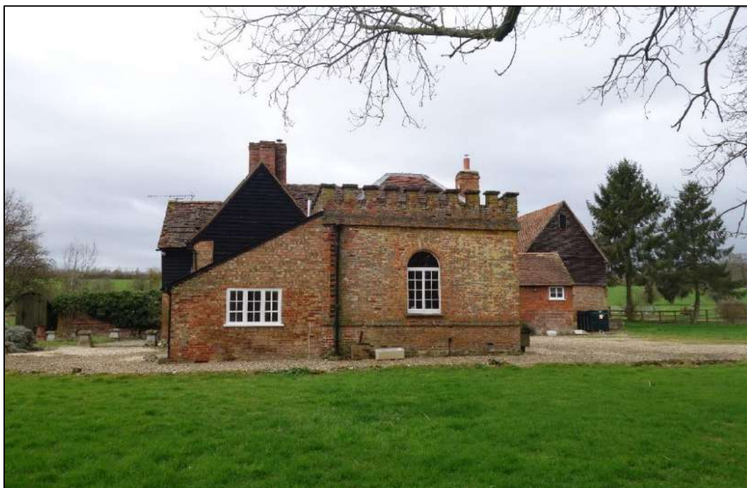
Plate 9: View looking W showing late 18 th century castellated brick extension to E end of farmhouse
