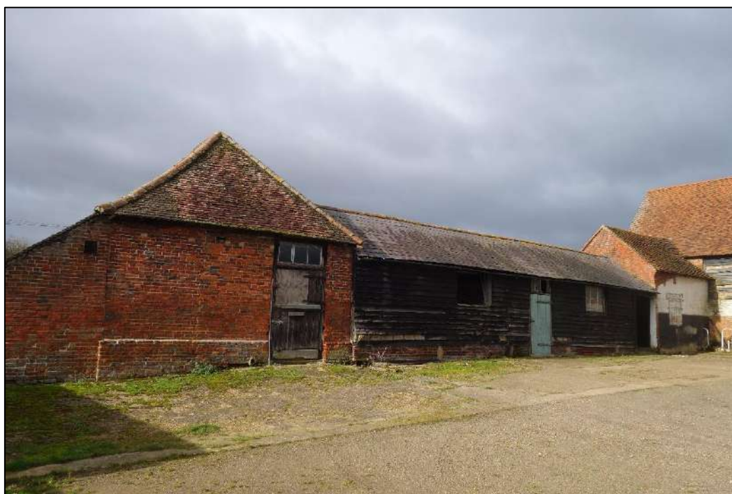
Plate 61: Oblique view looking NW showing front (E-facing) elevation of West Stables
