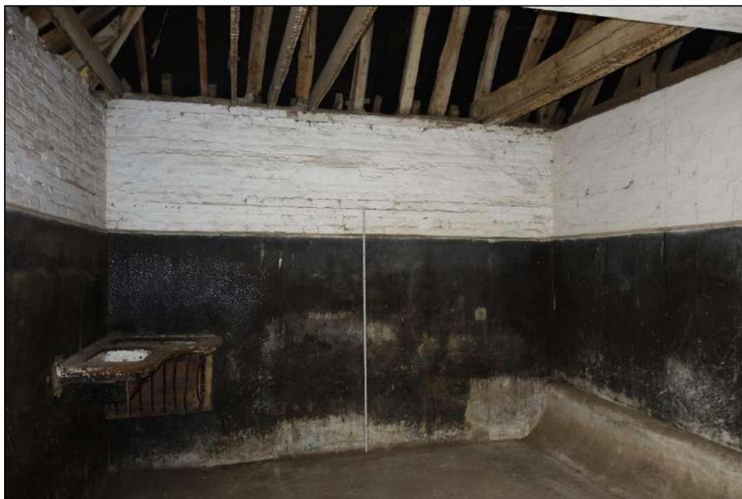
Plate 72: View looking S within eastern compartment of stable block at S end of West Stables
