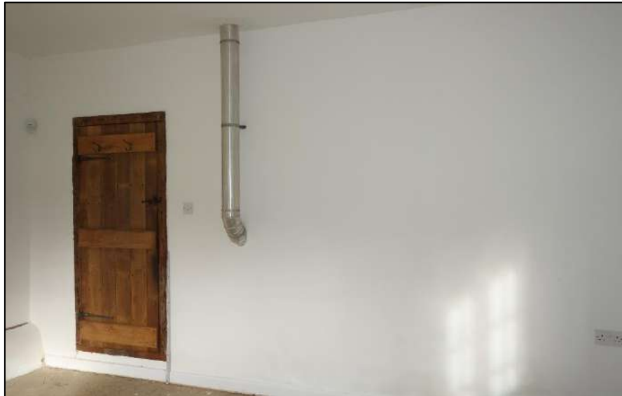
Plate 32: View looking NW towards N wall of Dining Room showing modern flue to right of doorway
