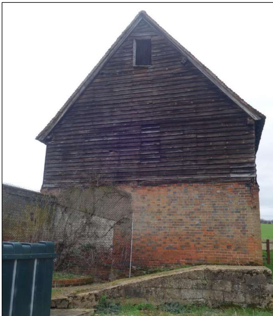
Plate 54: View looking W showing E-gable end of Barn with outline of demolished early 20 th century lean-to structure visible to left of picture
