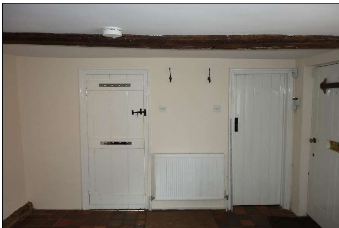
Plate 24: View looking S showing partition wall at S end of Scullery with doorway to living room to left and cloakroom to right of picture
