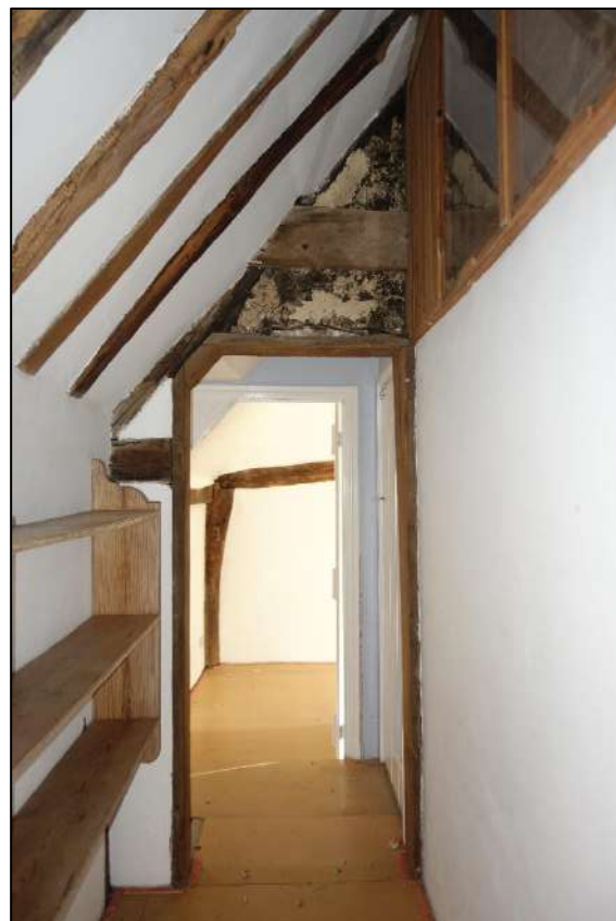
Plate 34: View looking E along first floor corridor showing exposed timber-framed panels
