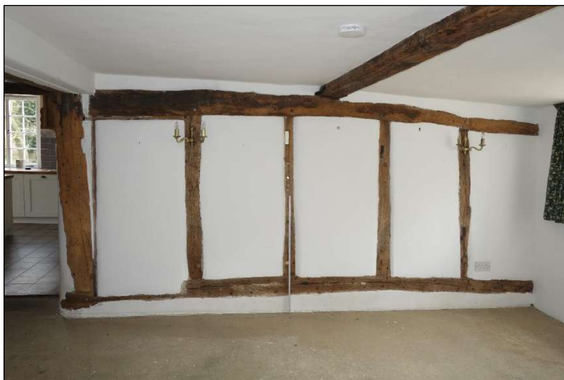
Plate 19: View looking E within living room showing exposed timber framed panels in E wall
