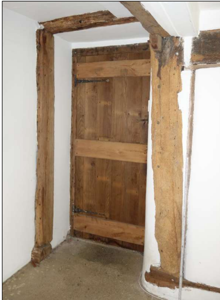
Plate 22: View looking NE towards doorway from living room to Kitchen with moulded skirting at base
