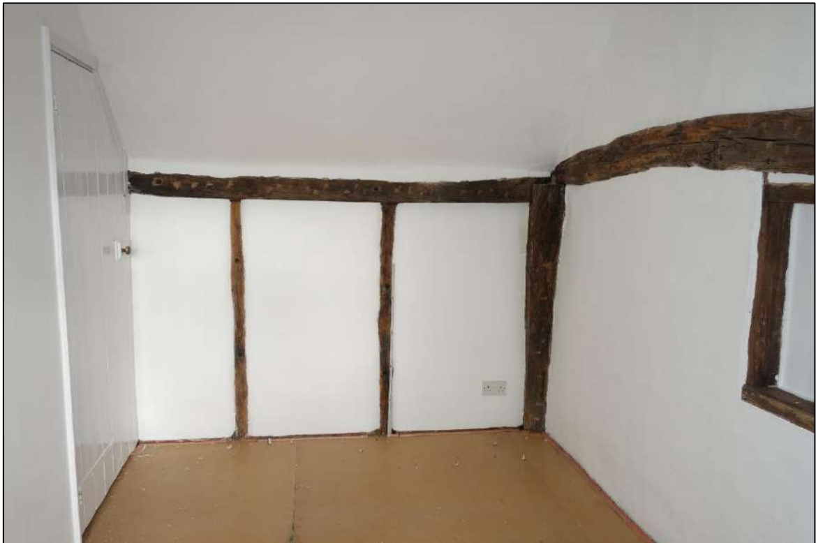
Plate 48: View looking N showing thin-scantled timber-framed panels with plaster infill in N wall of Bedroom 3
