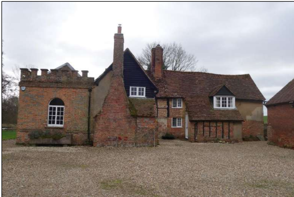
Plate 4: View looking S towards principal N-facing elevation of farmhouse
