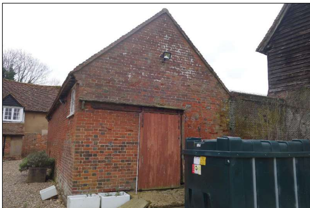
Plate 76: View looking SSW showing N-gable end of East Stables with modern sliding door inserted for dairy
