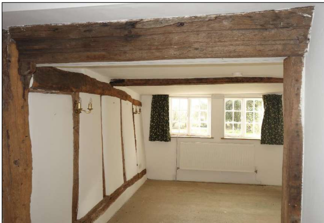
Plate 18: Internal view of living room looking S showing moulded beam supported by vertical timber posts
