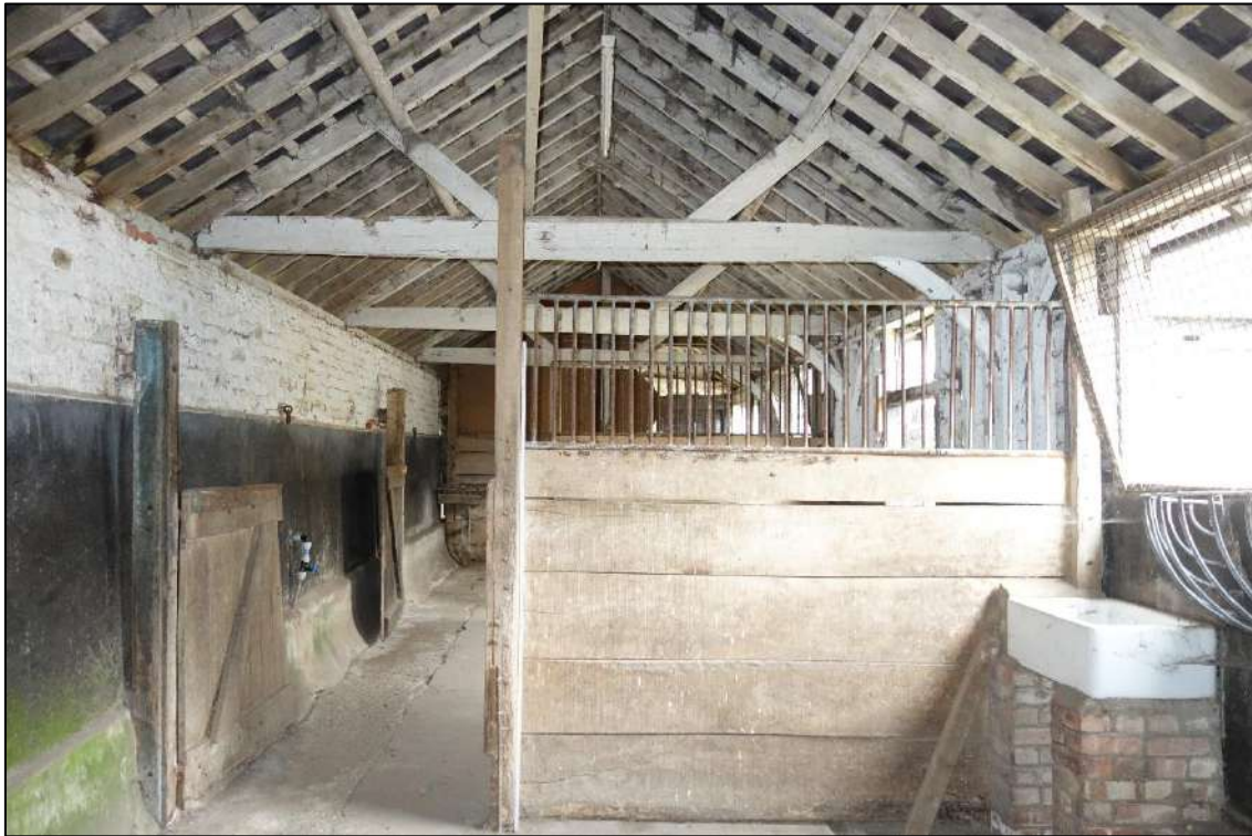
Plate 69: View looking N within weatherboarded stable range showing detail of open-truss roof structure
