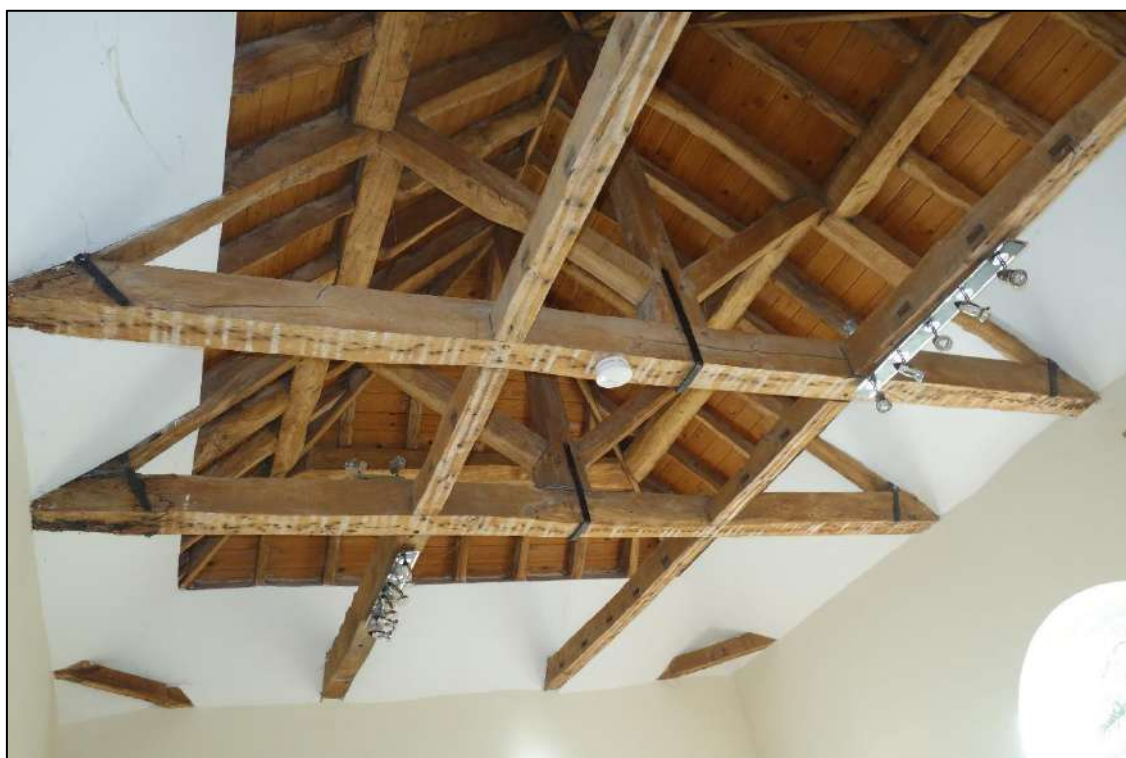
Plate 29: View showing kingpost roof trusses and ceiling beams in Kitchen
