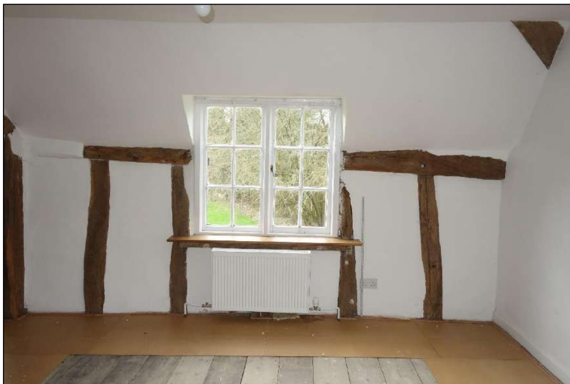
Plate 38: View looking S showing casement window inserted within earlier timber-framed panels in S wall of Bedroom 1
