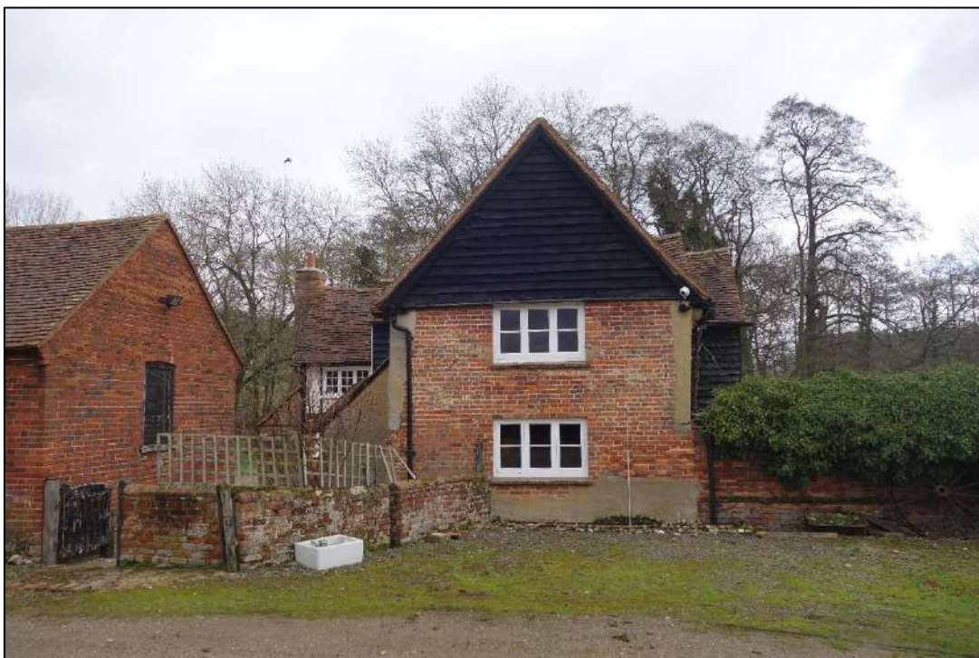
Plate 7: View looking E showing W-facing gable of farmhouse with mullioned casement windows
