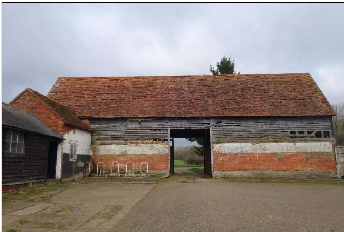
Plate 52: View looking N showing S-facing elevation of Barn with partially whitewashed brickwork and indentations for former lean-to outbuilding
