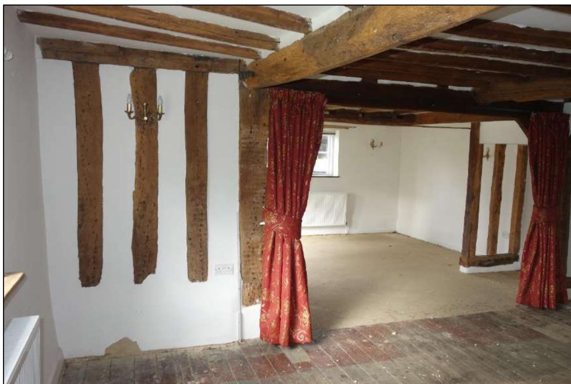
Plate 16: View looking W showing close-studded timber framed panel in W wall of southern bay of sitting room
