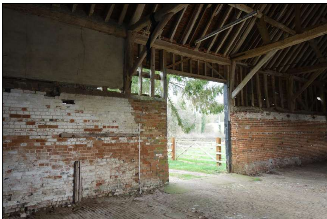
Plate 58: Internal view of Barn looking NE showing N entrance flanked by whitewashed brick walls and brick cobbled threshing floor to right
