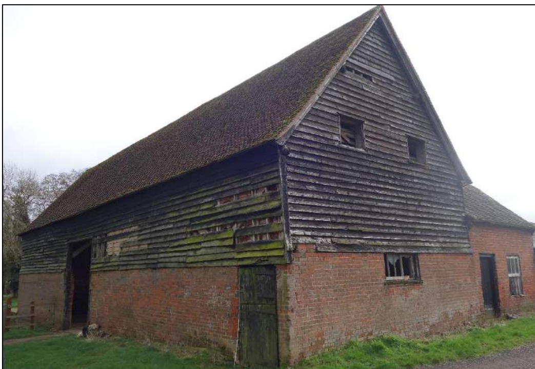
Plate 53: View looking SE showing weatherboarded W-gable end of Barn with doorway to chaff room and granary at W end of barn and single storey annexe with pitched roof (tack room) to right of gable
