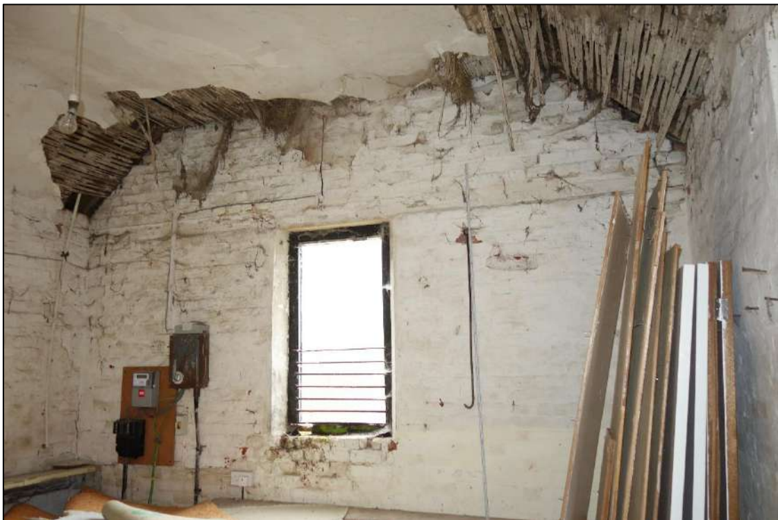
Plate 77: View looking SE showing compartment at S end of East Stables with coved plaster ceiling
