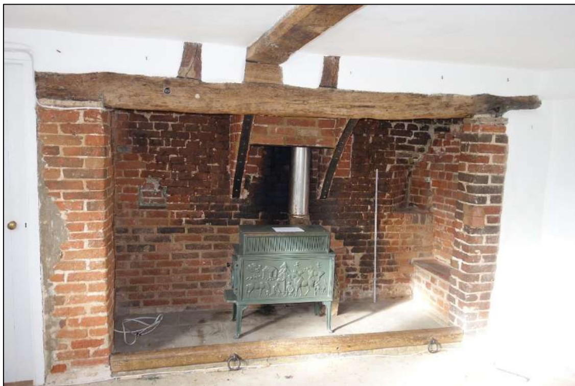
Plate 20: View looking W showing brick fireplace with inglenook in W wall of living room
