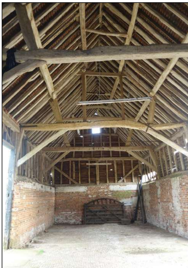
Plate 55: View looking E showing central and E portion of Barn with queenpost roof structure
