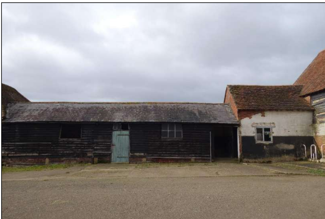
Plate 62: View looking W showing single storey gabled brick 'tack room' with adjoining weatherboarded stable range to left
