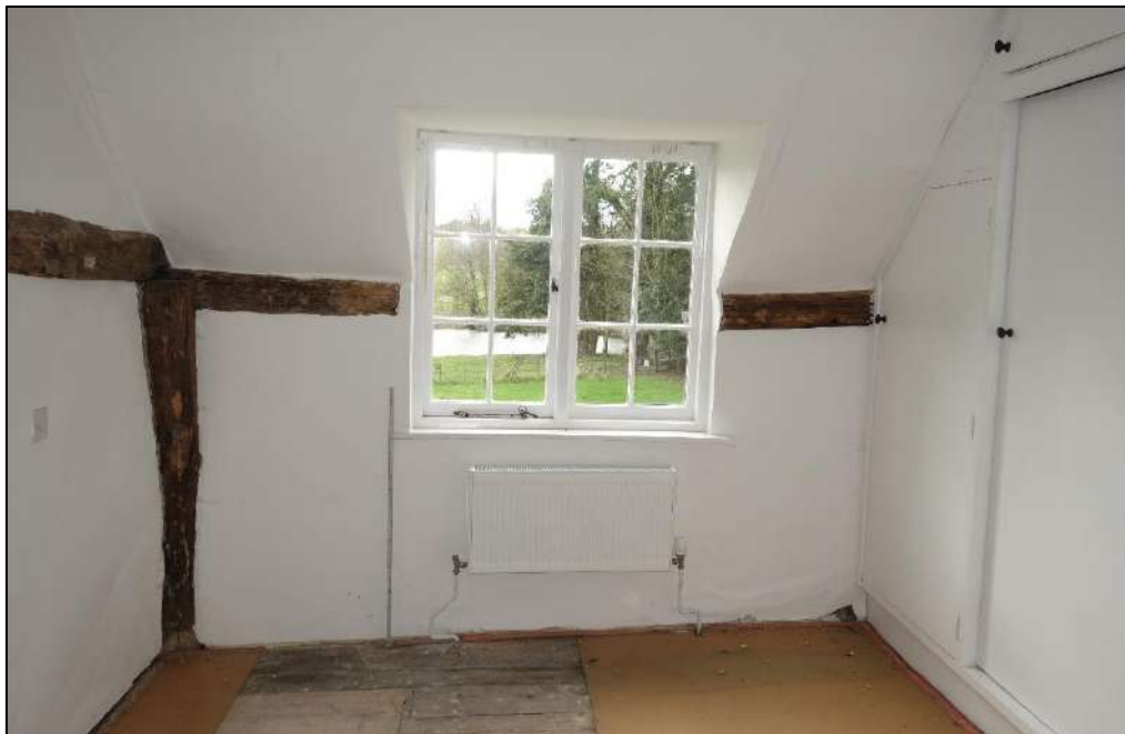
Plate 47: View looking S showing interior of S portion of Bedroom 3 with exposed floorboard beneath window
