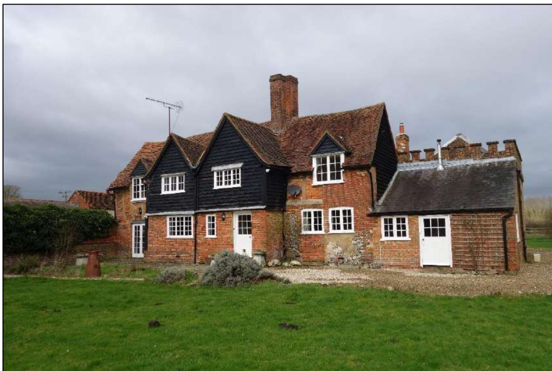
Plate 2: View looking NW showing rear of farmhouse with outbuildings to W
