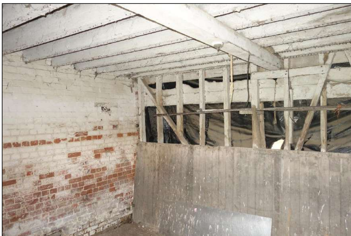
Plate 60: View looking NE showing interior of chaff room below granary at W end of Barn
