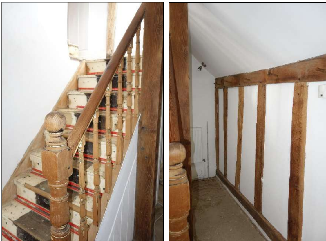
Plate 10: Internal view looking towards staircase in entrance vestibule in farmhouse, leading up to the first floor
