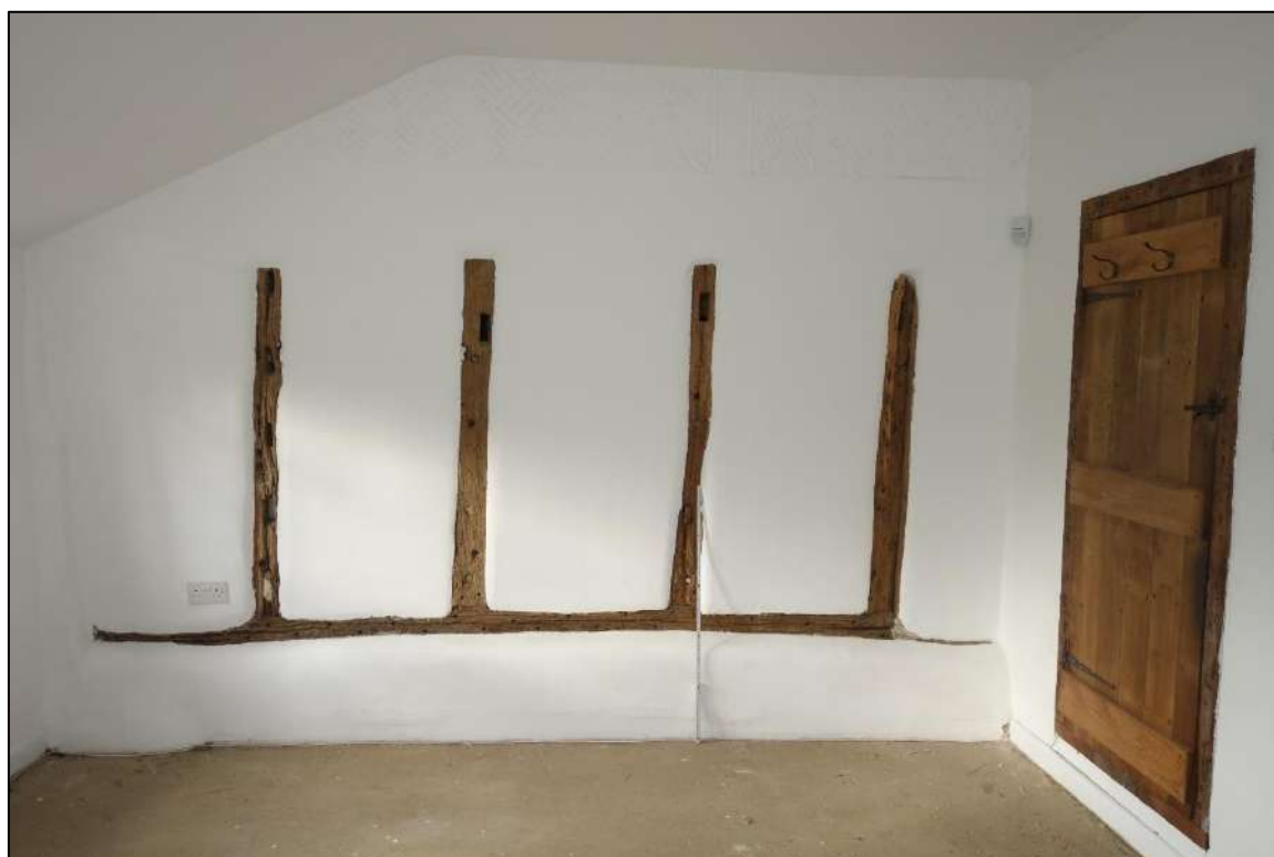
Plate 31: Internal view looking W showing W wall of Dining Room and sunken floor level
