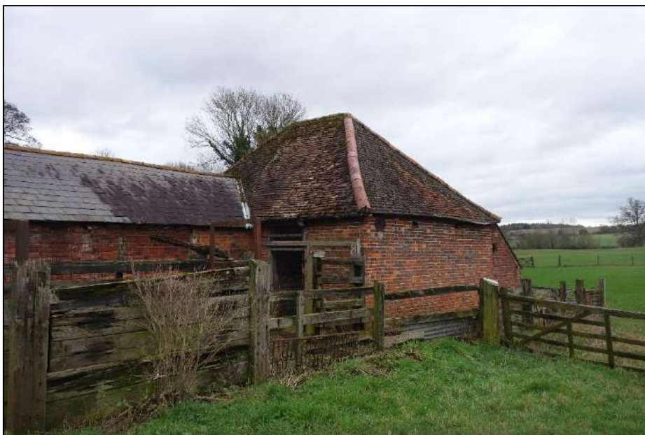
Plate 65: View looking SE towards two-bay stable block with pyramidal tiled roof
