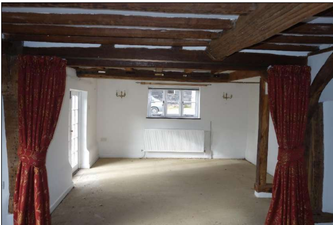
Plate 13: View looking W towards W end of sitting room with exposed roll moulded ceiling beam (in foreground) and casement window in W wall
