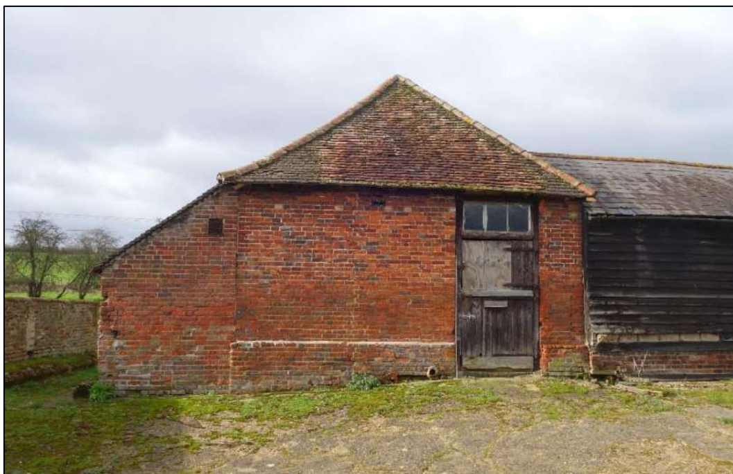
Plate 63: View looking W showing brick stable block at S end of West Stables with pyramidal tiled roof and attached lean-to piggy to S
