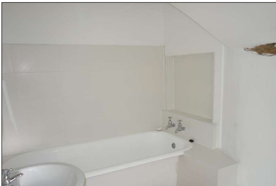
Plate 41: View looking NE showing partition walls to N and E of bath suite in bathroom to SE of Bedroom 1
