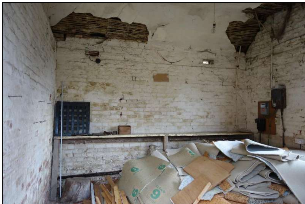
Plate 78: View looking W showing interior of southern compartment with shelving and nails in wall for harness
