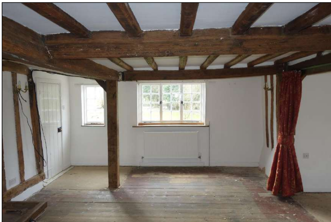
Plate 15: View looking S towards southernmost bay of sitting room, showing exposed ceiling beams and floorboards
