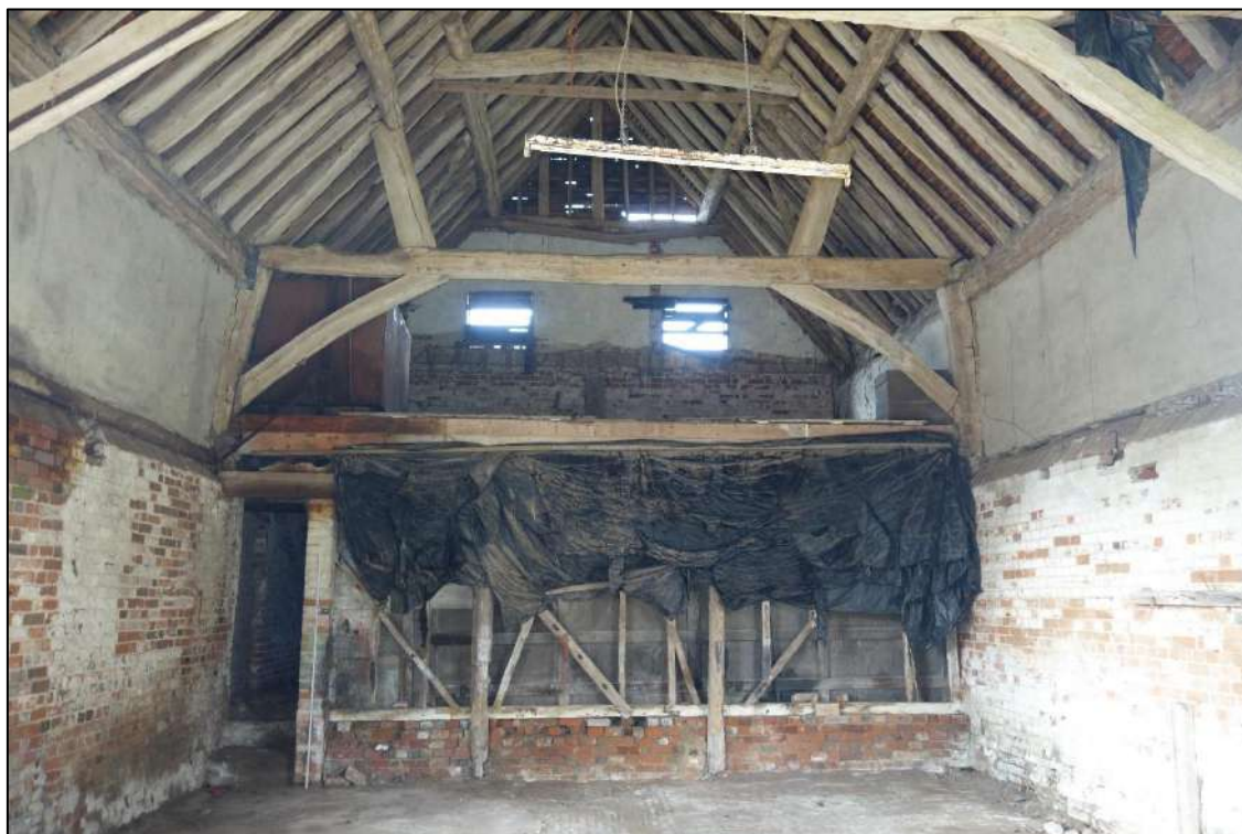
Plate 59: Internal view showing brick and timber-framed partition at W end of Barn for chaff room and granary loft above
