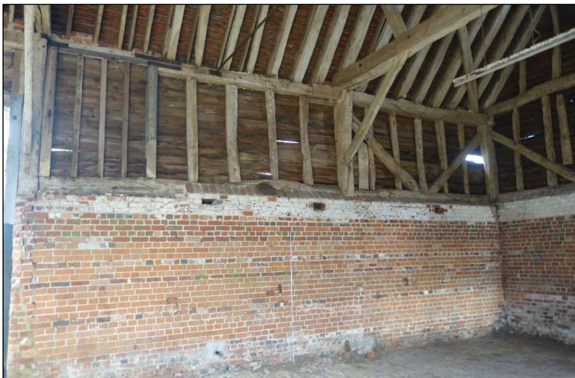
Plate 57: Internal view looking NE showing partially whitewashed N wall of Barn with timber framed panels resting upon brick walls
