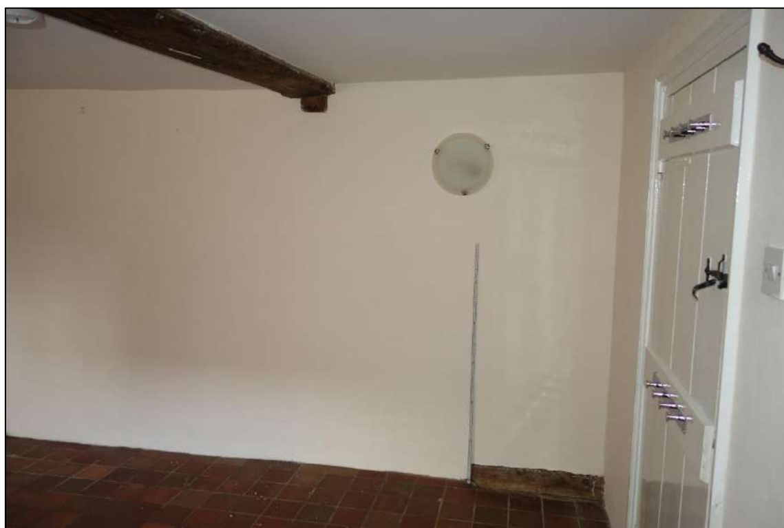
Plate 26: Internal view showing E wall of Scullery with exposed ceiling beam and remnant of moulded wallplate (to bottom right of picture)
