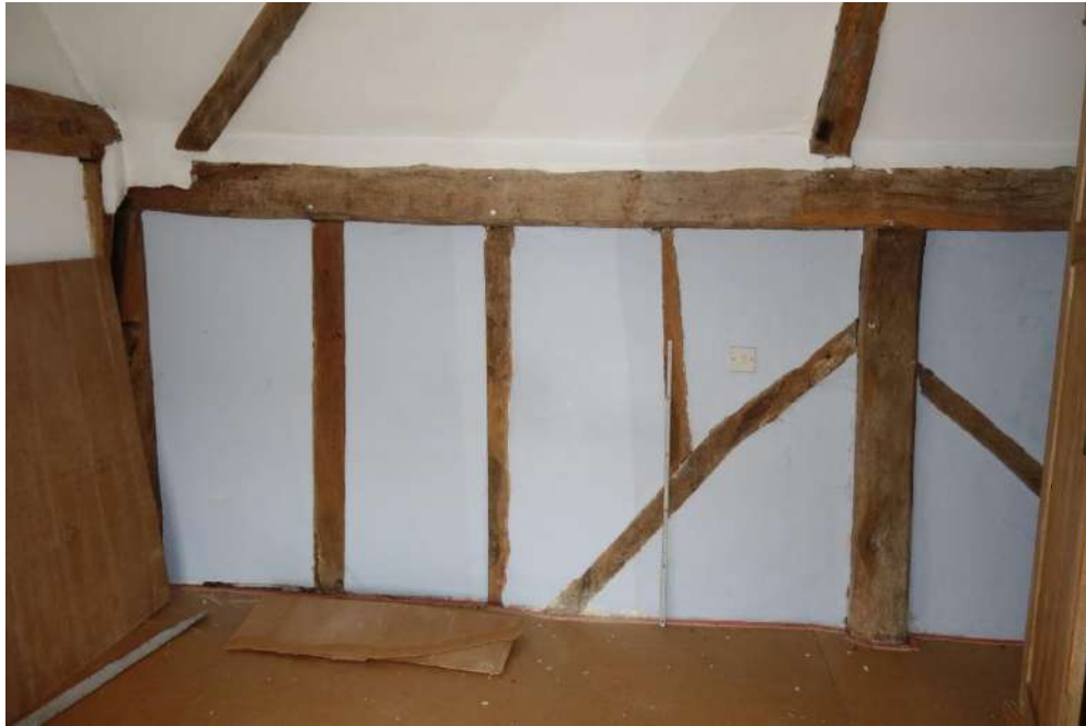
Plate 46: Internal view looking E showing E wall of Bedroom 2 with exposed timber framed panels with vertical wall-posts and vertical and diagonal studding
