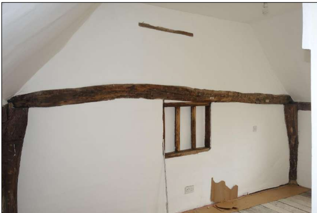
Plate 49: View looking E showing E wall of Bedroom 3 with exposed timber-framing and blocked three-light mullioned window
