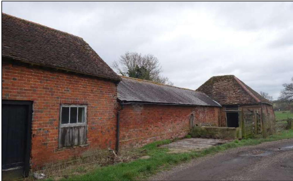
Plate 64: Oblique view looking SE along rear elevation of West Stables towards late 18 th -early 19 th century stable block with pyramidal roof at its S end
