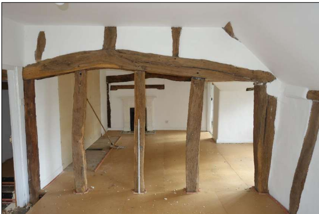
Plate 36: Internal view looking E within W half of first floor bedroom showing curved tie-beam and studded partition
