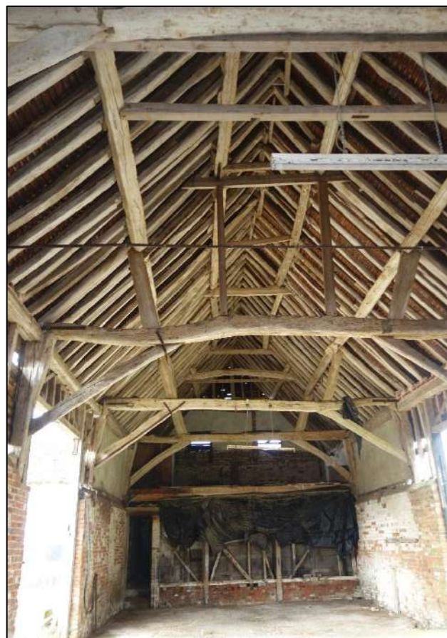
Plate 55: View looking E showing central and E portion of Barn with queenpost roof structure
