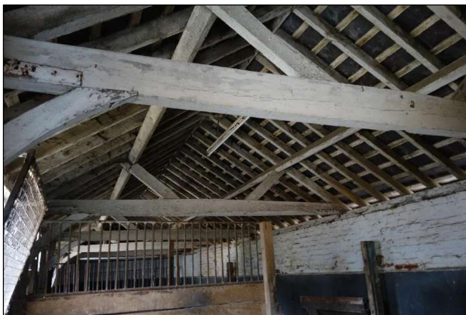
Plate 67: View looking S along central portion of three-bay stable range, showing loose box partitions and roof trusses
