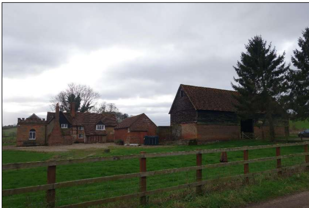
Plate 1: General view of farmhouse and outbuildings looking SW from trackway
