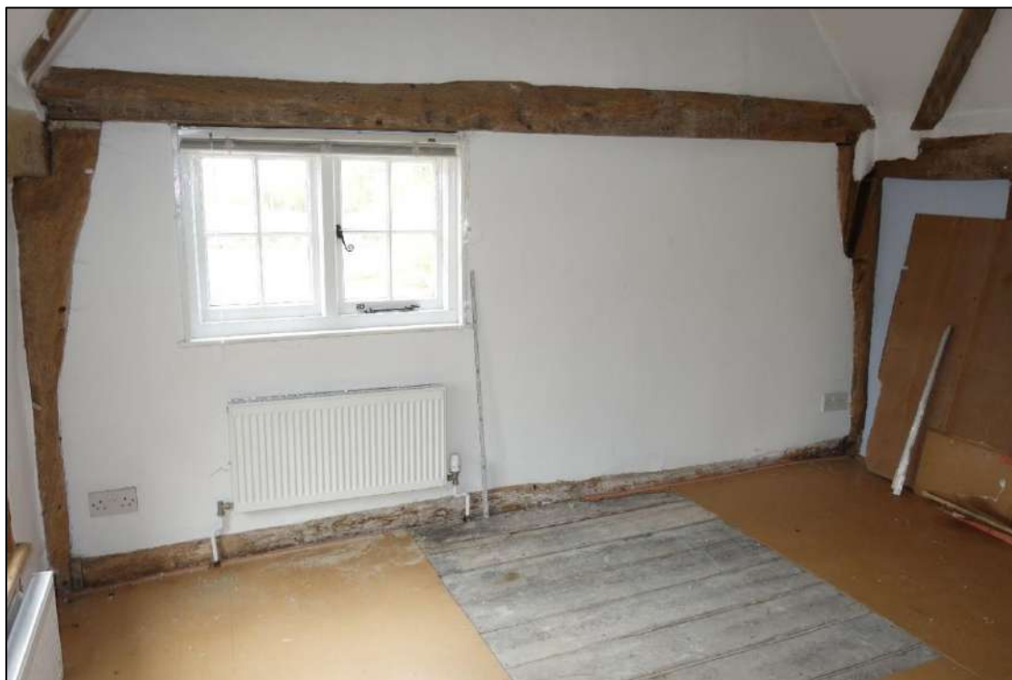
Plate 44: View looking N showing N wall of Bedroom 2 with exposed timber wall plate and flanking jowelled posts
