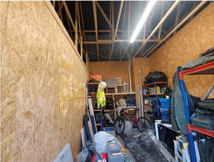
Fig 17 – barn rebuilt in sterling board and off the peg trusses
