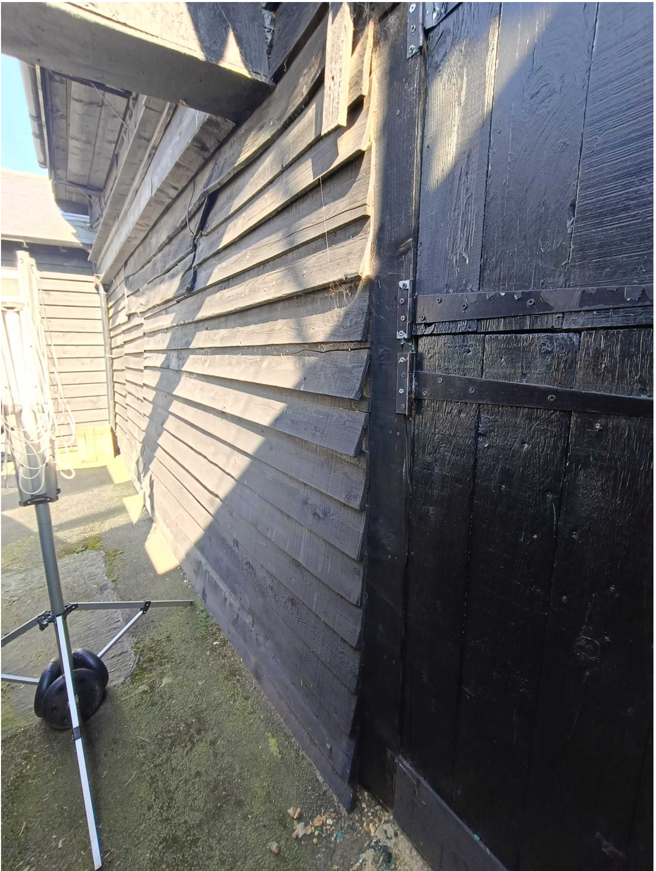
Fig. 15a – possible C18 timber section remaining at junction of SW wall and NW structures
