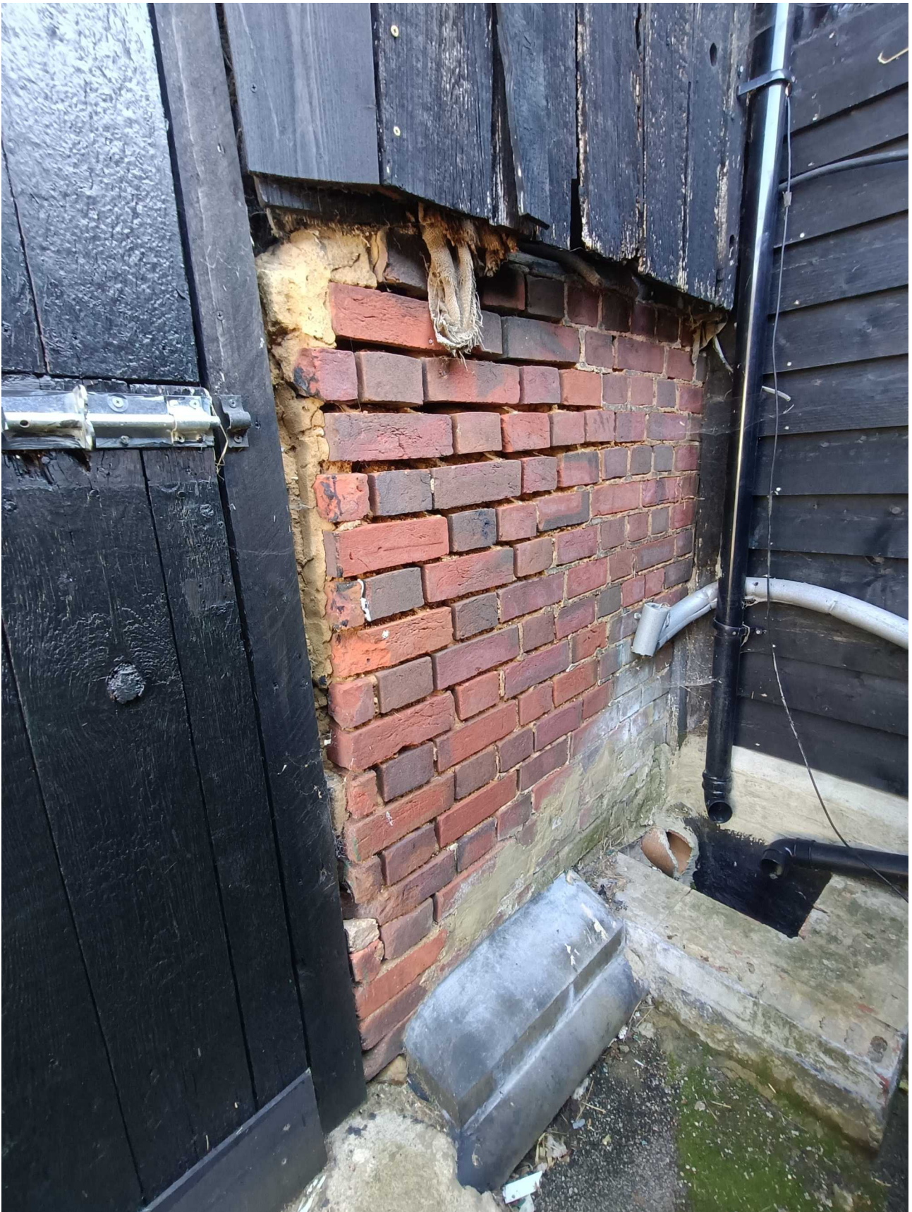
Fig 15b – the rest of the SW wall in late C19 monk bond brick with piers concealed on inside
