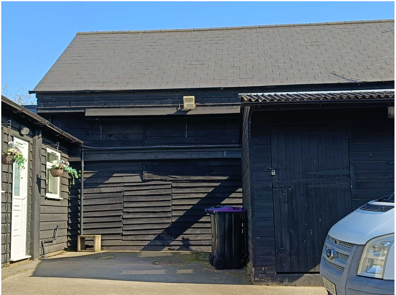
Fig 18 – smooth lines of new structure rising above small retained section on SW wall
