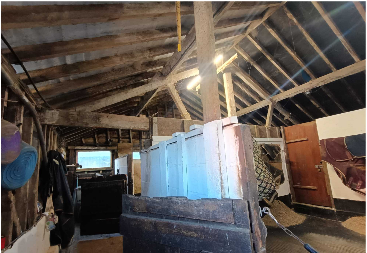
Fig 16 – Interior of stables attached to NW elevation of barn. Rafters of different scantling. Later partitions
