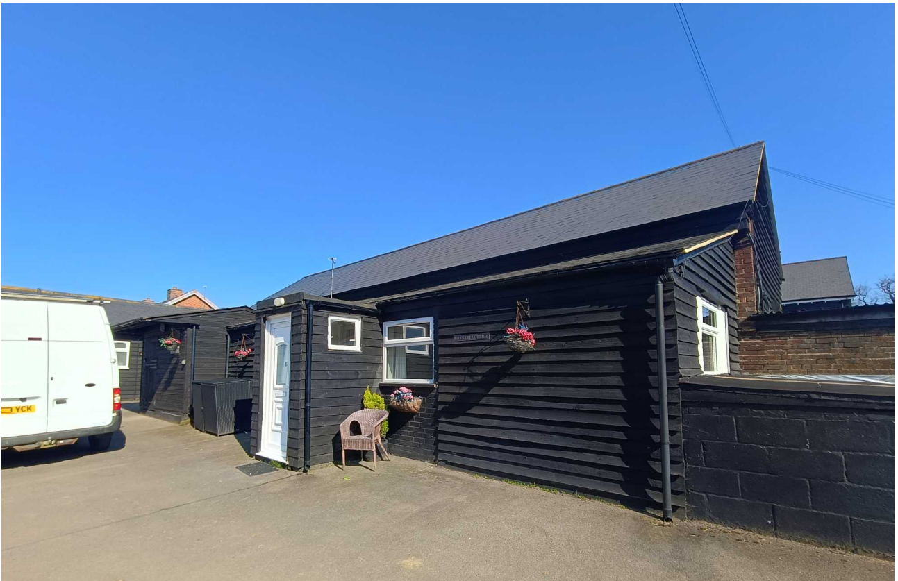
Fig 15c 1950s extension in front of continuing brick wall. New barn rises above. Barn house beyond.
