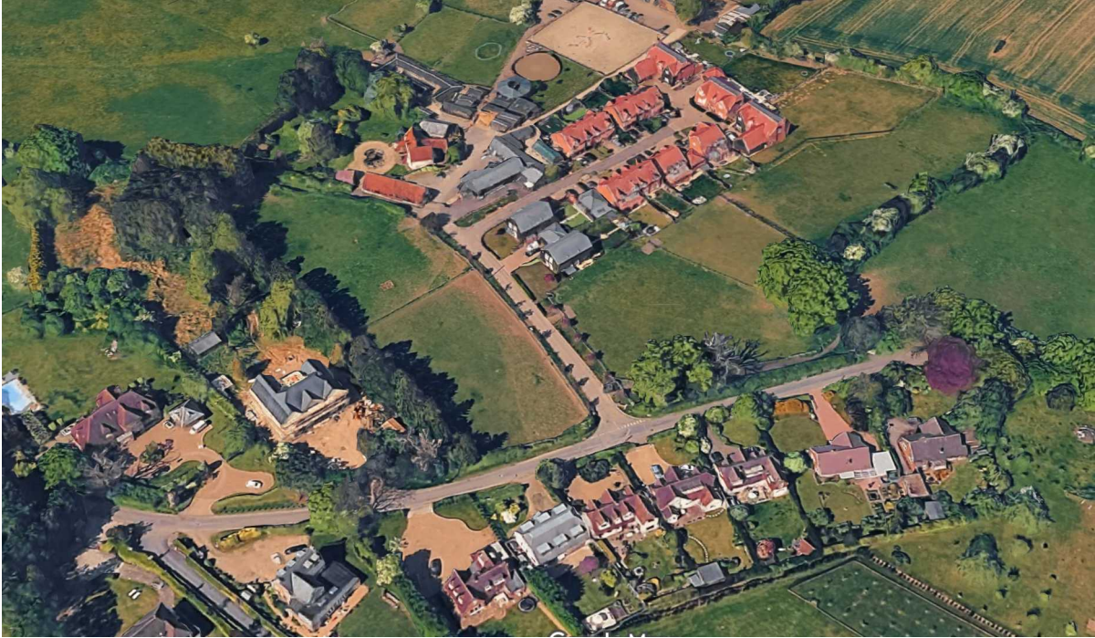
Fig 22- The drive showing 1930s houses to east, 1920s deep plot to south (right) and 'Stables' to north
