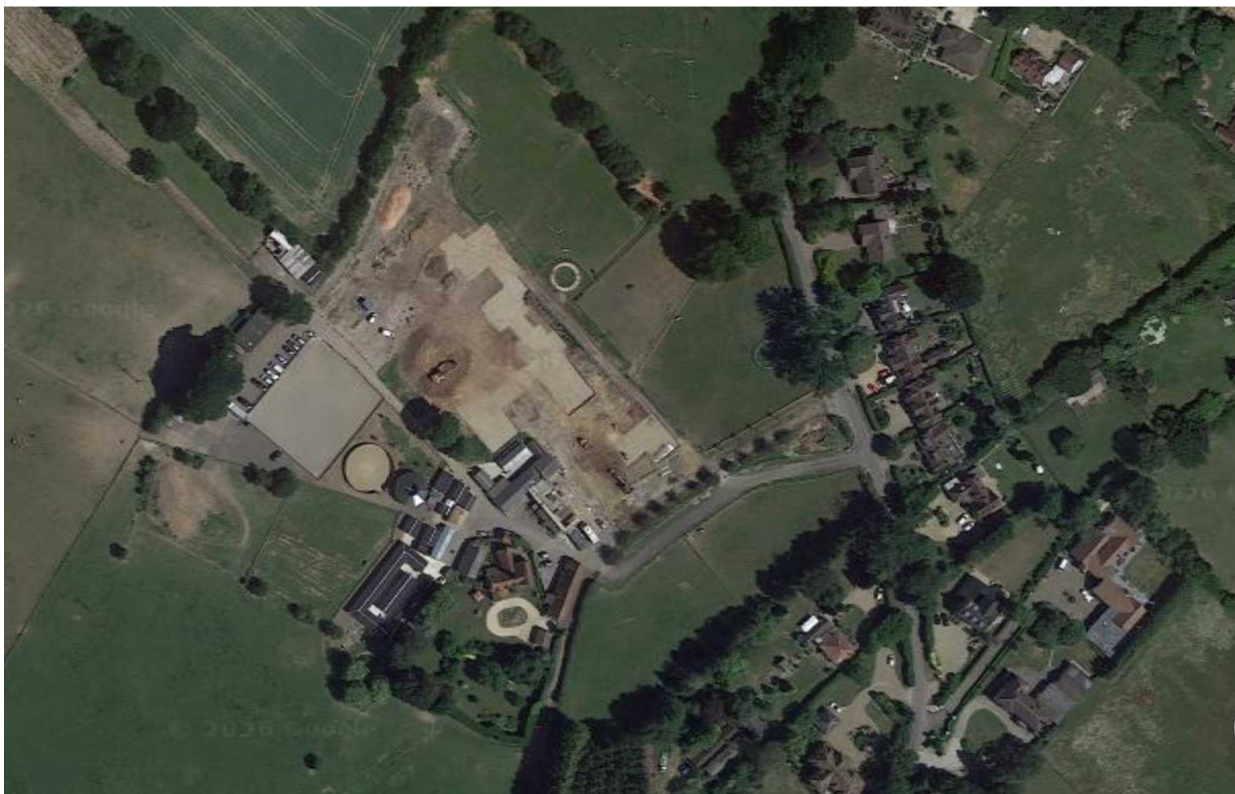
Fig 11 – 2018 aerial showing barn razed to the ground
