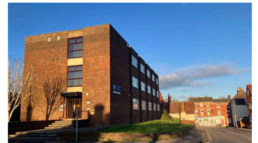
5. No.1 Wratten Road East office block
