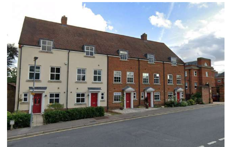
3. No 1-5 Old Charlton Road Row Houses (Courtesy of Google Maps )
