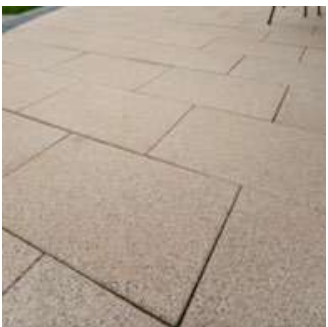
Terraces and paths – Light coloured slabs laid in staggered pattern.
