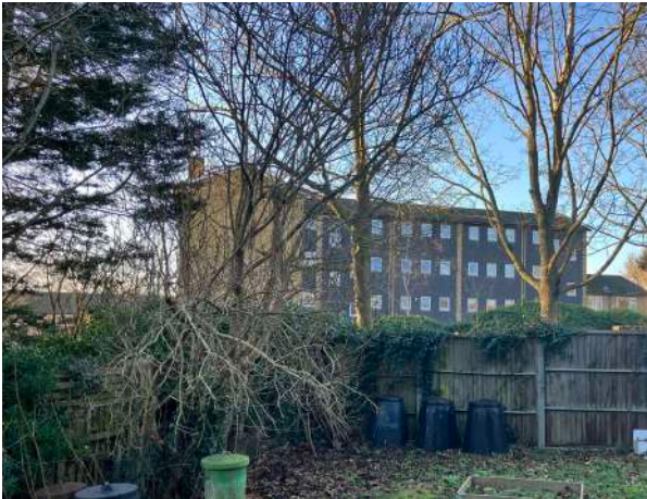
E Silverdale House view from garden
