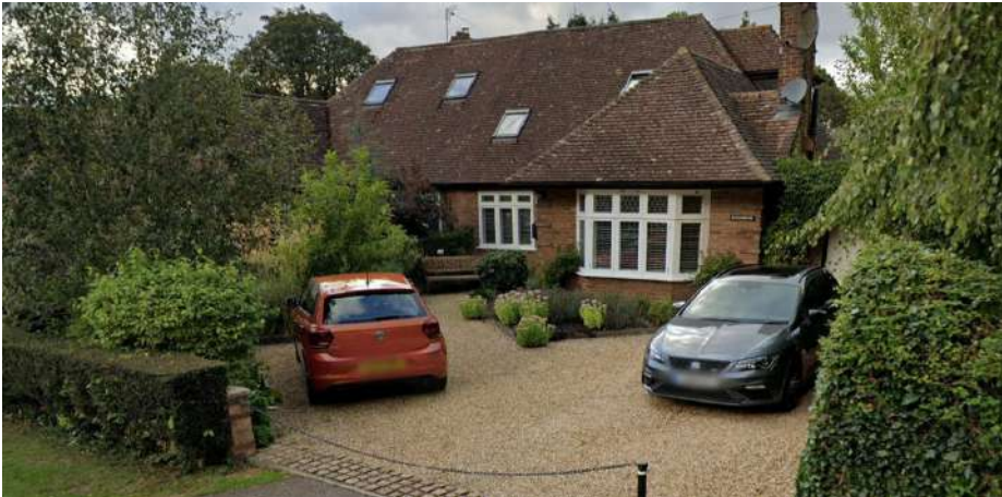
D Birchwood House frontage (Courtesy of Google Maps)
