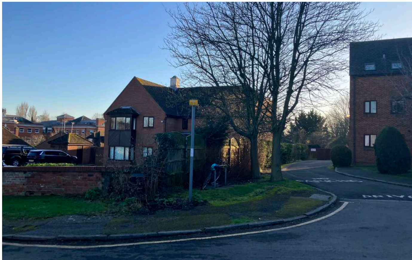
Indicative view 7 (Existing)- From the front of the Grade II Listed Wrattan House looking south
