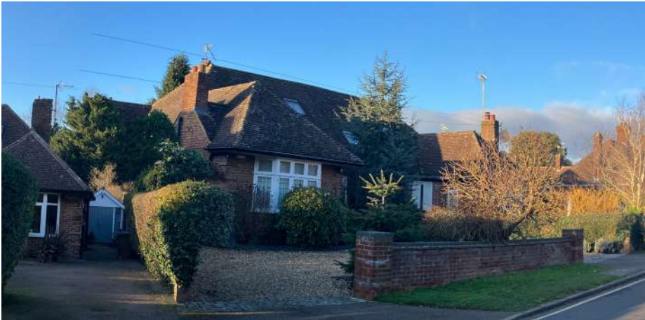
C Willow Close House frontage
