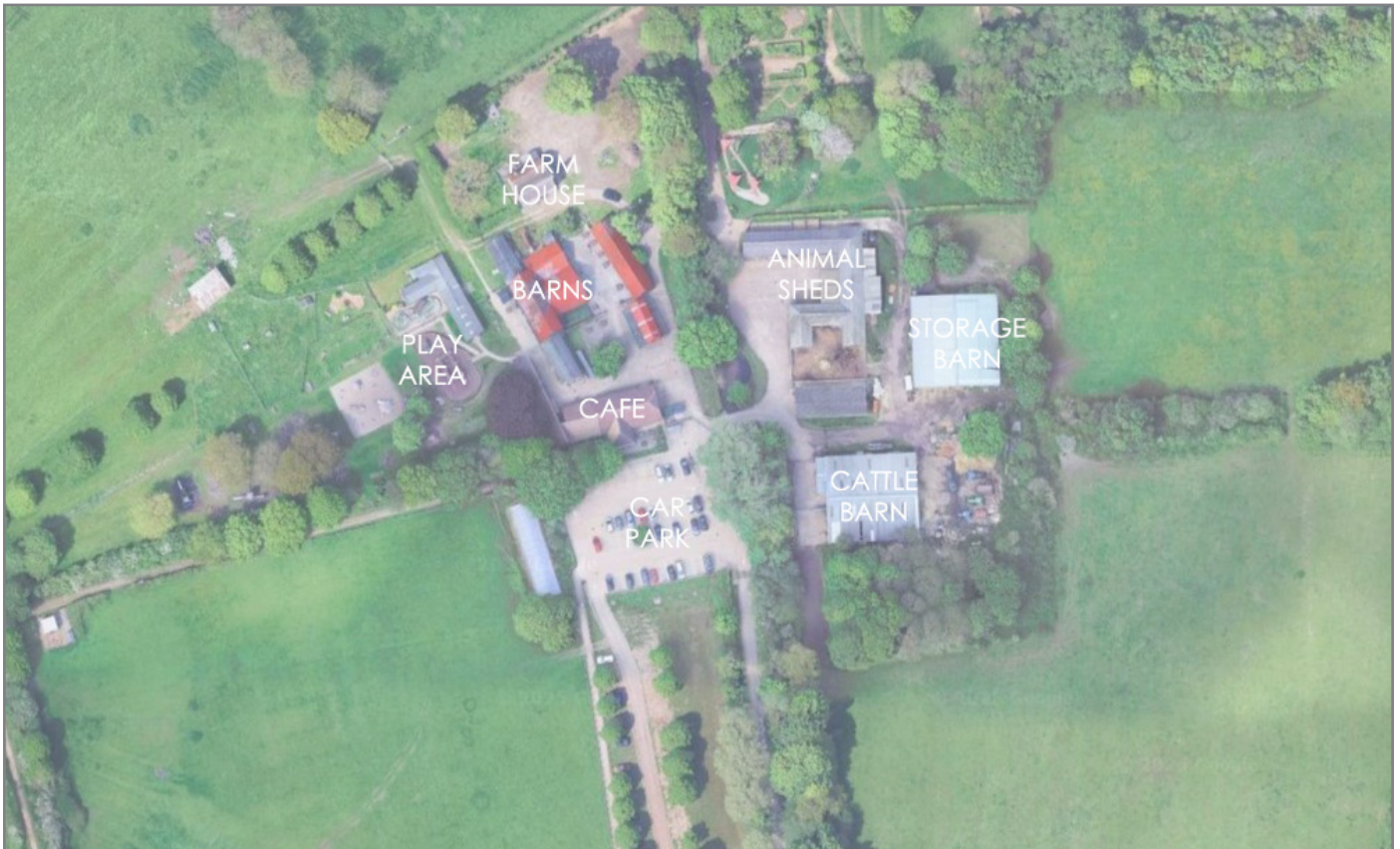
Standalone Farm: Google Earth view of the farm buildings
