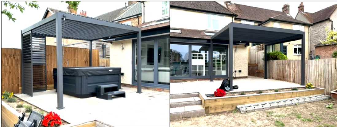
View of pergola on eastern side of patio
