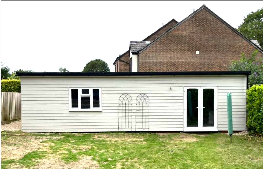
Enlarged outbuilding in rear garden currently under construction
