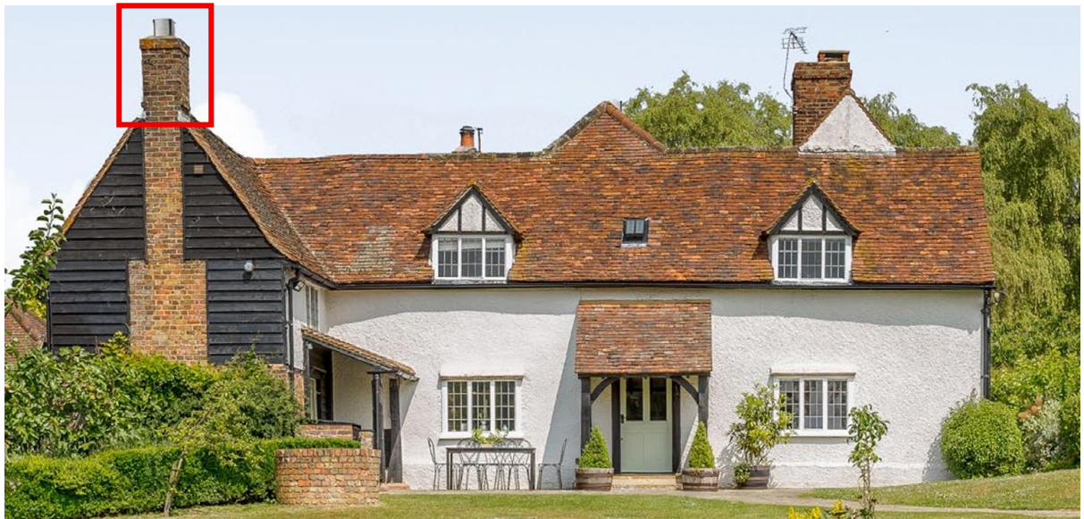
Figure 1 - Existing House showing Chimney under consideration
