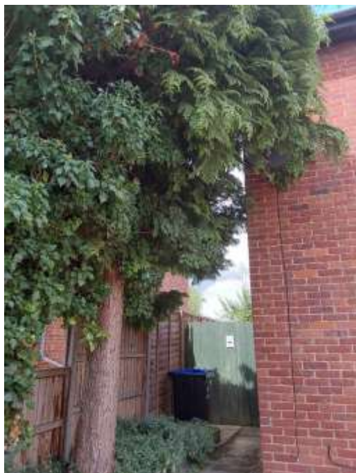
Plate 1: T001 and its proximity to the building.
