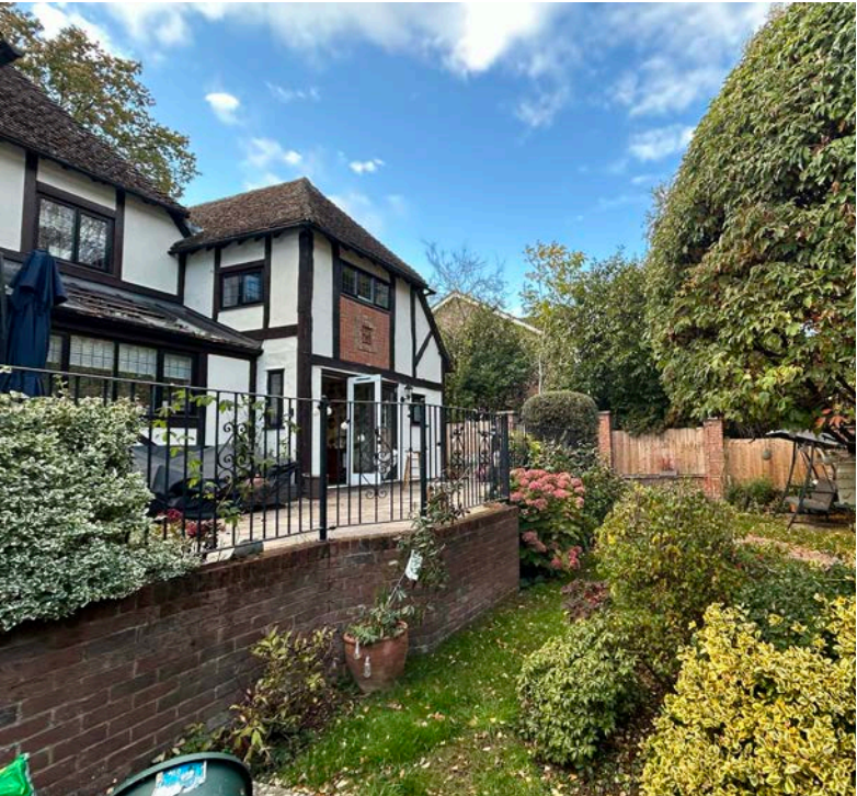
Rear side -- North-East Facade
