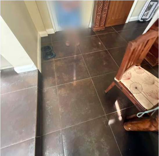
Ground Floor - single step between kitchen and dinning space
