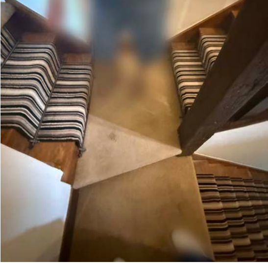
Multiple flights of stairs converge on one intermediate landing -- Convoluted circulation
