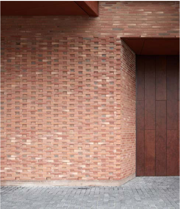
Munch Brygge Residential Complex Lund+Slaatto Architects
