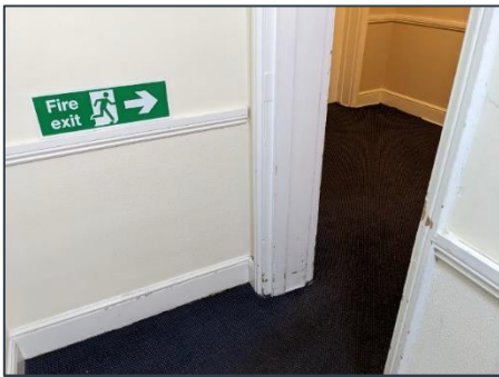
Sharp corners with narrow doorways
