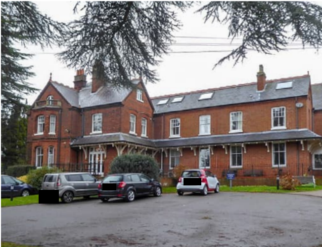
South façade of the original house, with 1980s extension to the right
