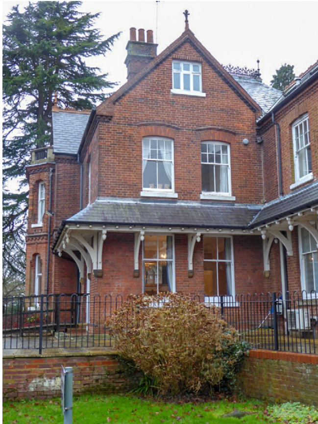
East façade of the original house
