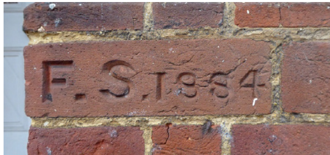
Inscribed brick to RHS of entrance porch
