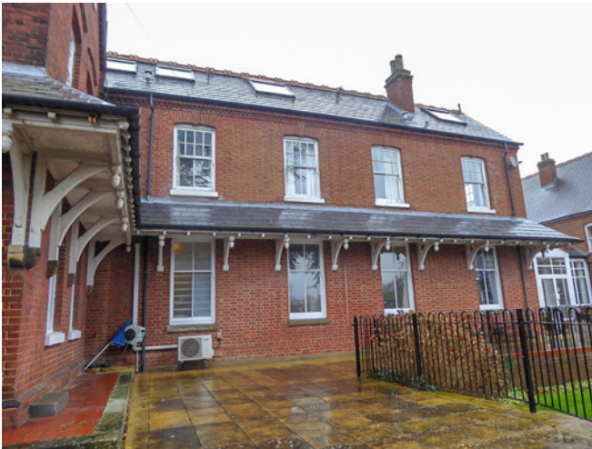
1980s wing: South façade
