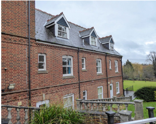
1990s wing: West façade
