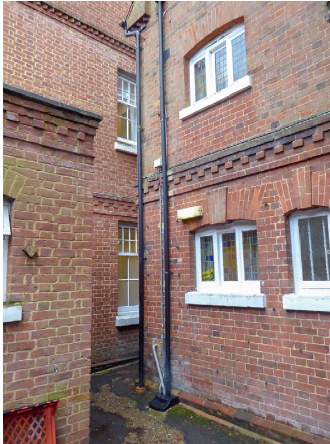
North façade of the original house (right), 1980s extension to the left
