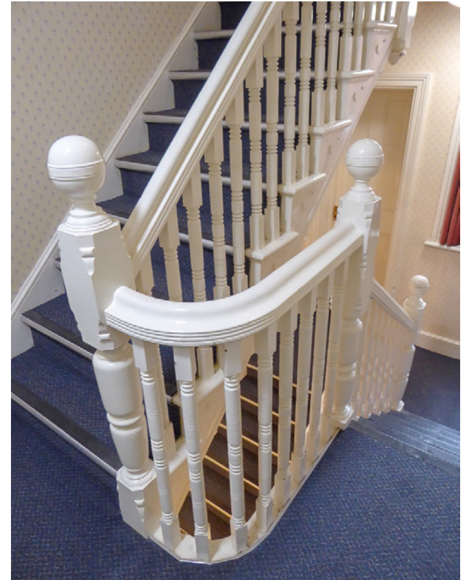
Main staircase at first floor level
