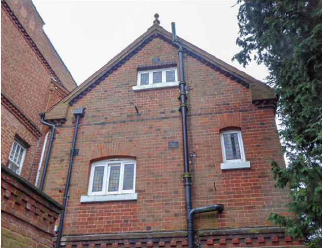
North façade of the original house: Upper floor, with 1980s extension to the left
