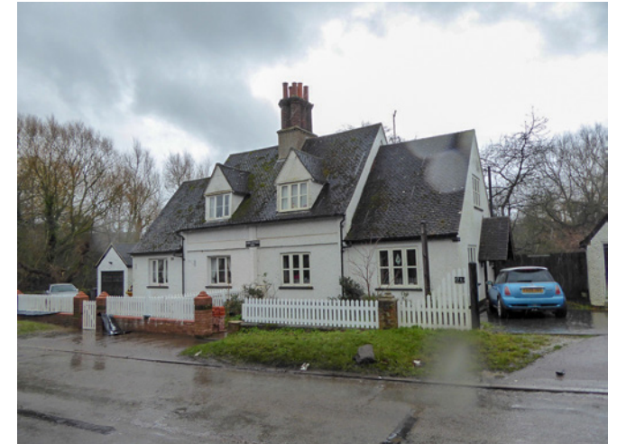
A pair of nineteenth-century cottages on the south side of Willian Road (not listed)
