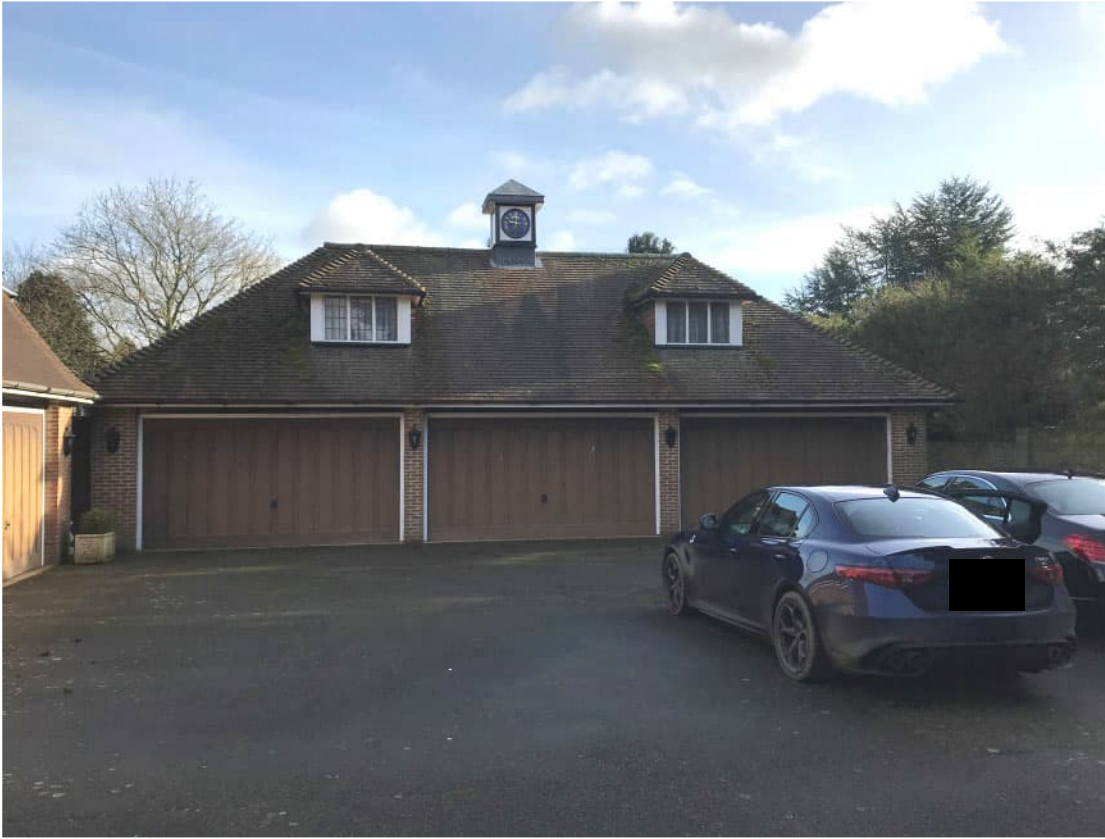
Photo 1 – North West Front of Garage Block
