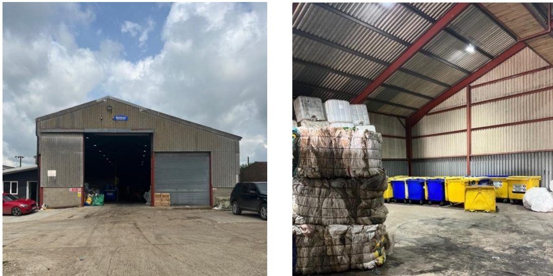
Figure 3.5 Exterior & Interior of B1 (images from 2023)
