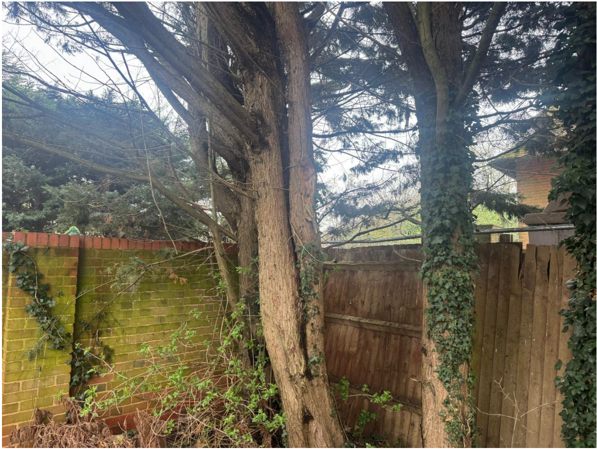
G1 – Leyland cypress group – Defective unions
