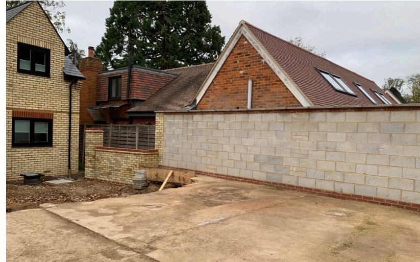
2 View from walled concrete yard towards neighbouring dwellings "Bury Lodge" and "Riverside Lodge"
