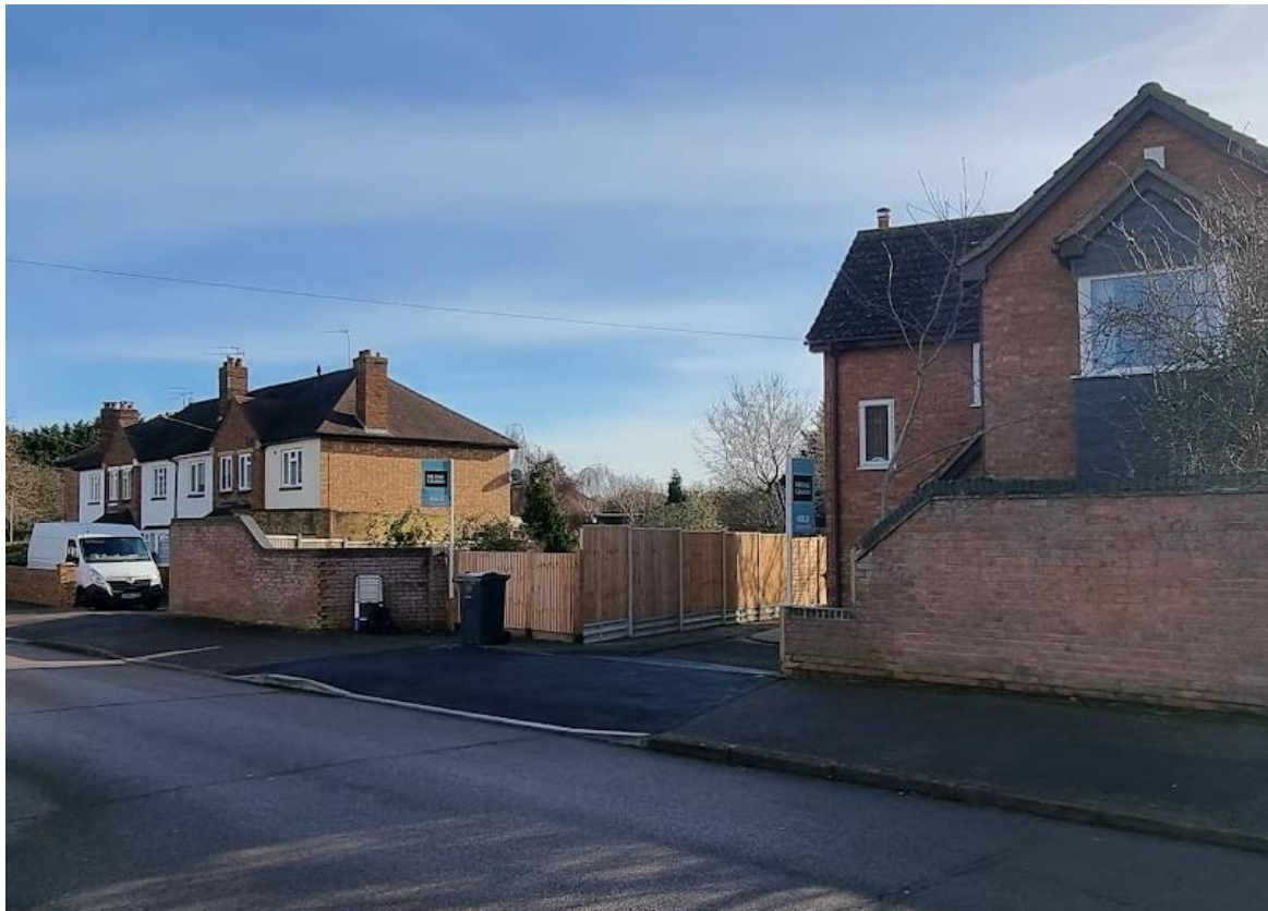
Looking East from Heathfield Road showing implemented crossover works.
