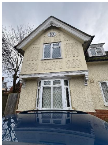
Existing front elevation windows with lead glazing
