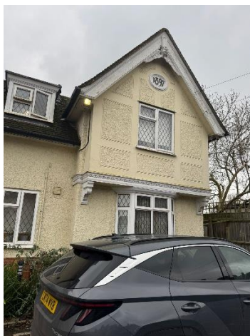
Existing front elevation windows with lead glazing
