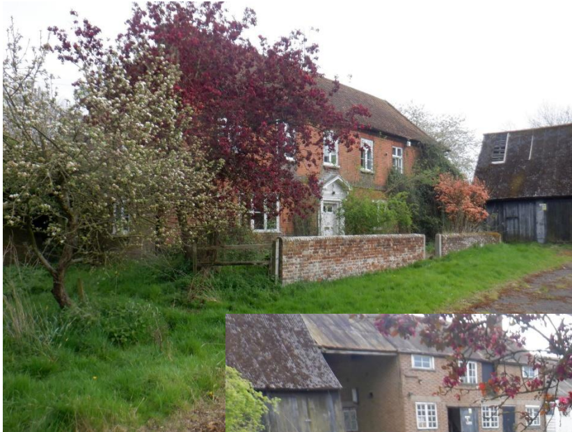
Front and North Elevations prior to implementation of permissions 23/00559/LBC and 23/00558/FPH
