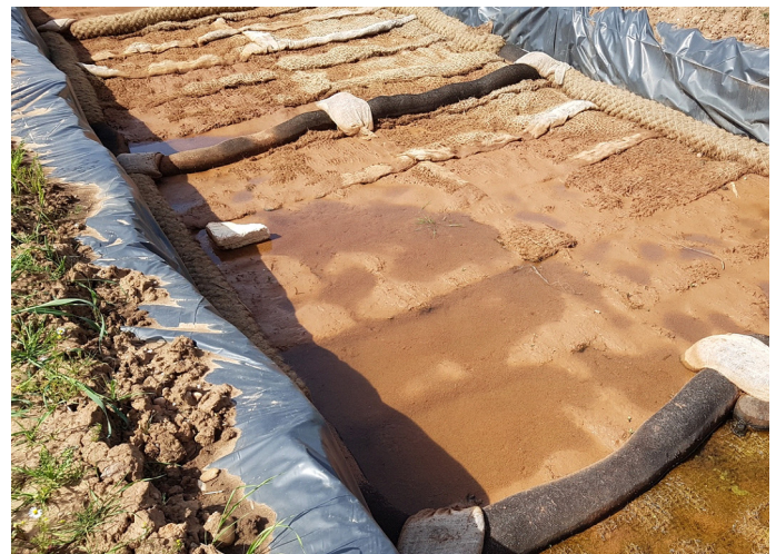
Deployed in Silt Capture Channels with Silt Wattles
