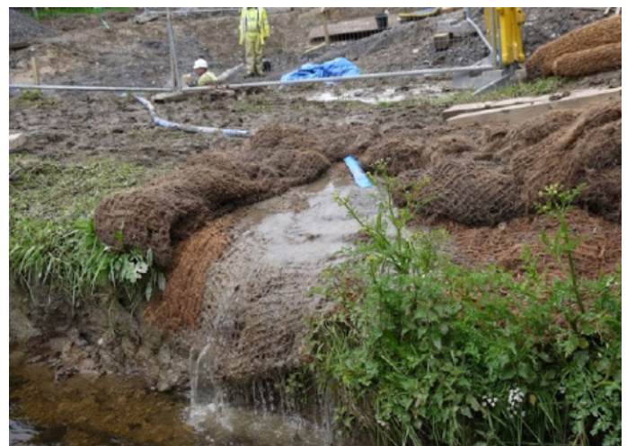
Deployed to treat muddy excavation water
