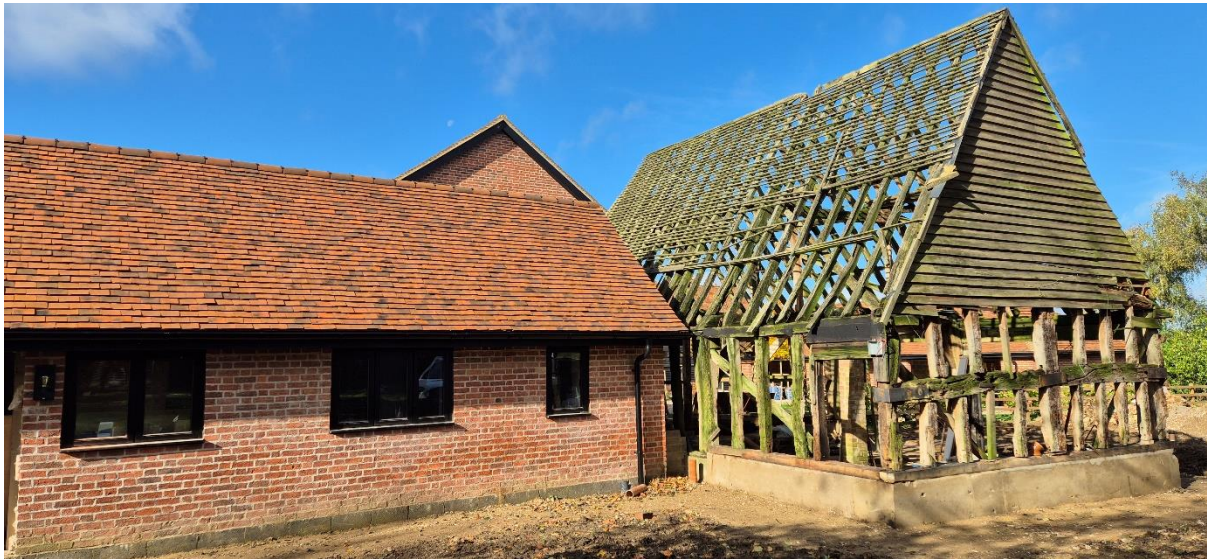
Listed barn from front.
