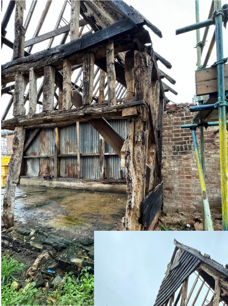
Photographs of linking wall on western elevation after commencement of permission 23/01999/LBC.
