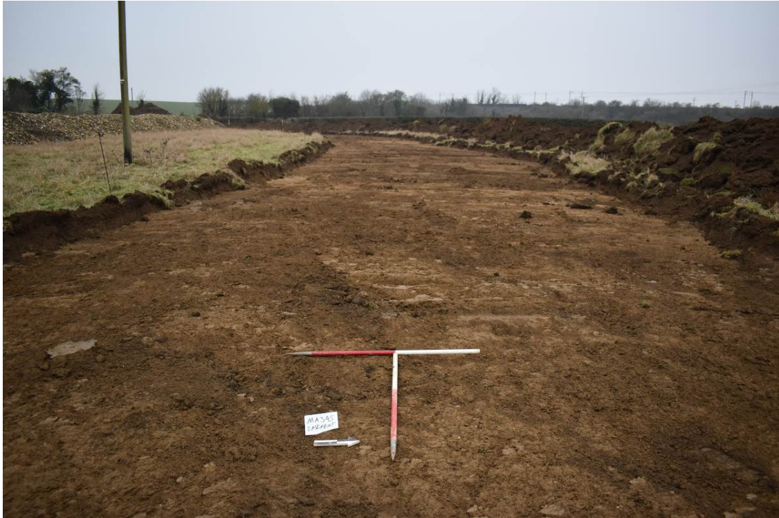
Plate 1: New access road – Looking West.
