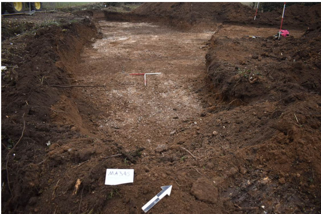
Plate 3: Bell mouth area – Looking Northwest.
