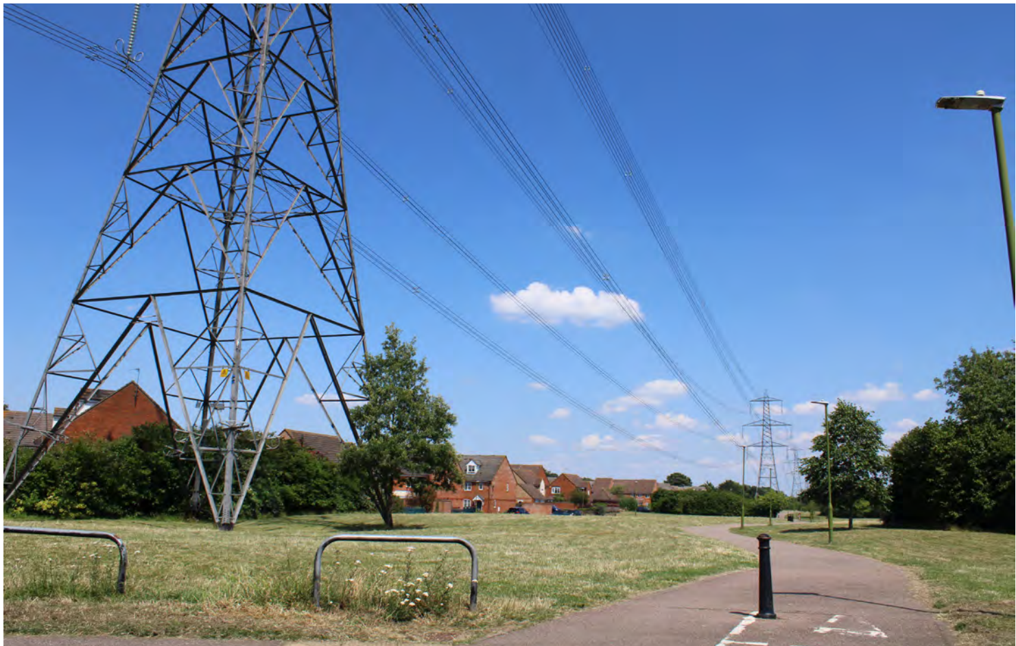
▲ Utility corridor utilised as leisure space
