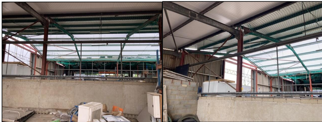
Photographs 8 - 9: Internal view
