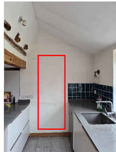
Figs. 04 & 05: the existing wall between the kitchen and library room (to be opened up). The previous doorway is outlined in red
