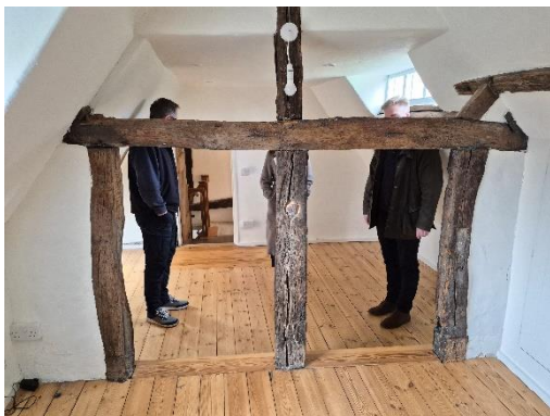
Figs. 07 & 08: The existing principal roof frame between Bedroom 3 and the new Dressing Room
