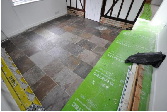
Fig. 12: Bedroom 1 existing floor
