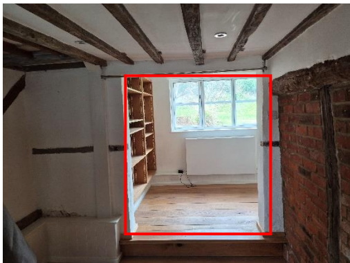
Fig 06. The existing opening between the library room and living room (to be closed up)
