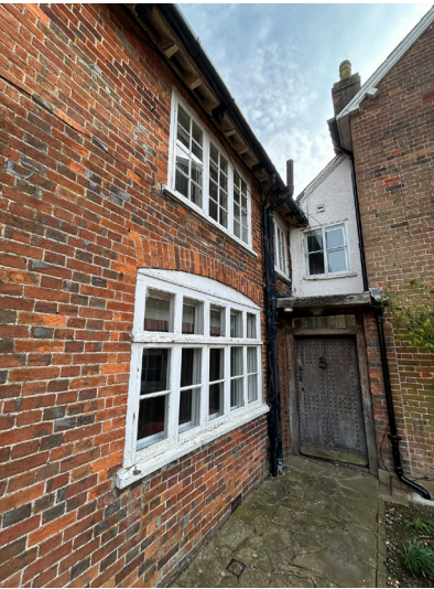
Photo of the principal elevation Georgian sash windows, 6 over 6 central sashes with 2 over 2 side sashes.
