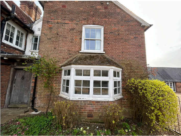
Photos of the north elevation at the rear of the house. Sitting adjacent to driveway access between front of house and rear yard and outbuildings.
