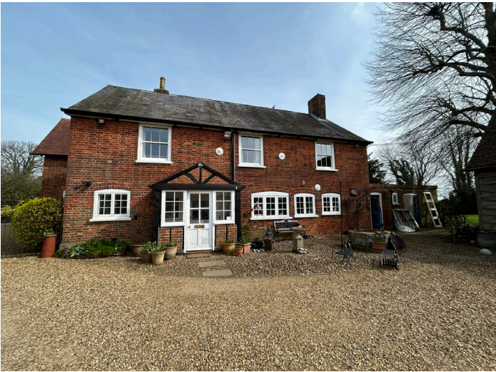
Photo of the rear elevation to the west, facing the yard opposite the grade II listed barn.
