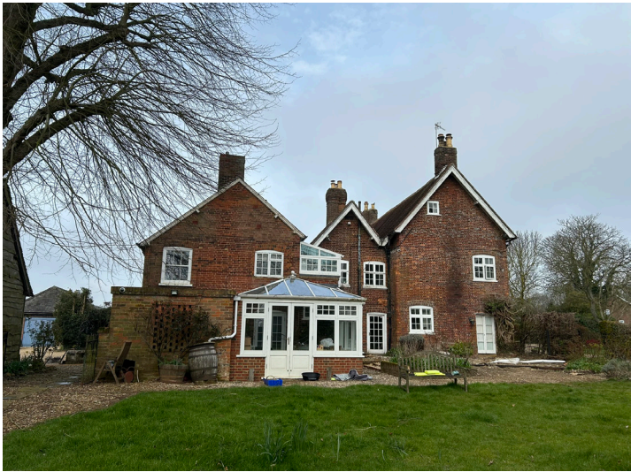
Photo of the south elevation, with modern conservatories.
