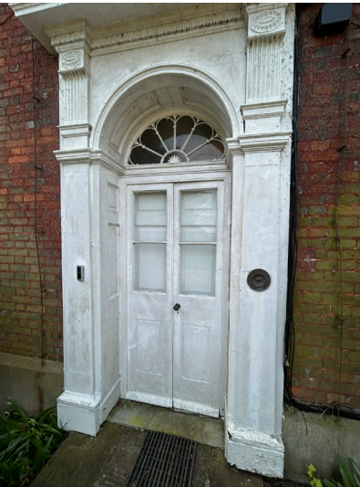
Photo of the principal elevation Georgian front door with canopy, decorative fan light over and outer French shutter doors.
