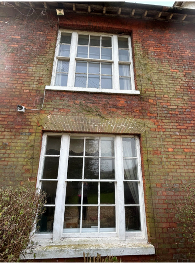
Photo of the principal elevation Georgian sash windows, 6 over 6 central sashes with 2 over 2 side sashes.
