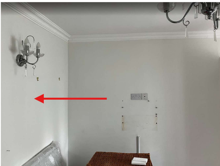
3.2.2 - Internal Wall View from Lounge
