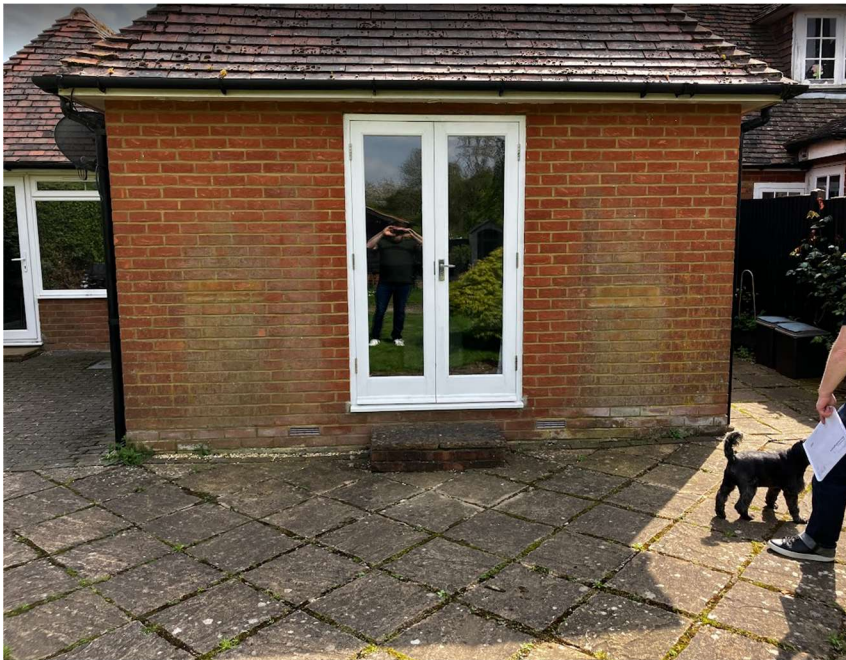
3.3.1 - Rear Doors - External View
