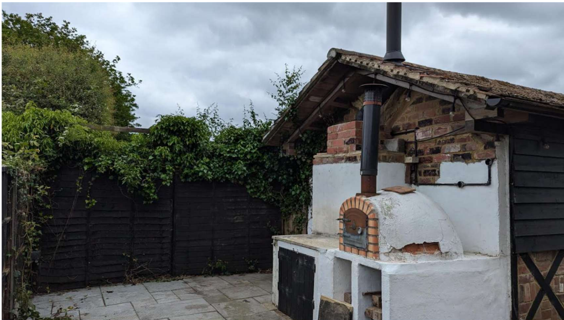
3.1.3 - Existing Garden Room - Rear View
