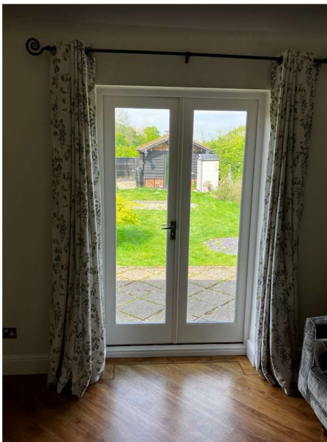
3.3.2 - Rear Doors - Internal View
