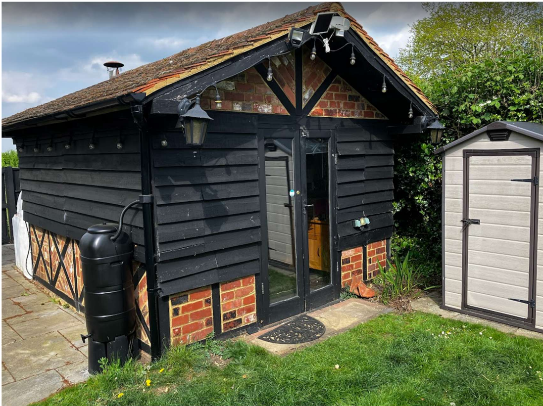
3.1.1 - Existing Garden Room - Front View
