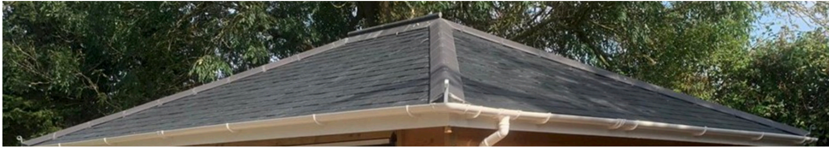
Slate roof, with black guttering
