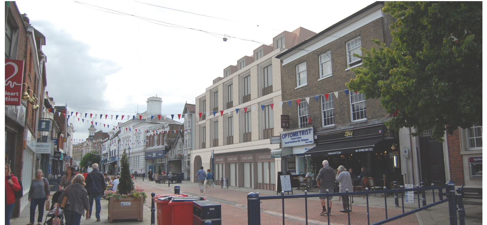
1. View from High Street taken facing south on High Street, Similar view to Conservation Area 2a, Key View 4
