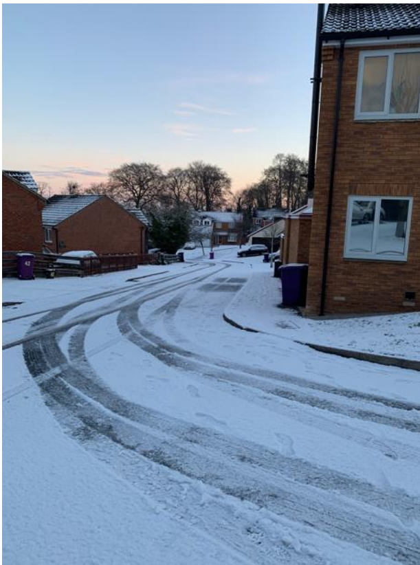
In poor conditions the road becomes a single lane track.
