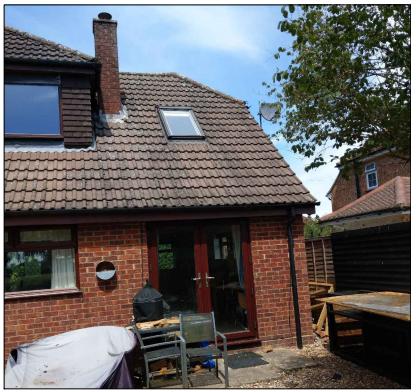
Existing / Proposed Rear View South East Corner
