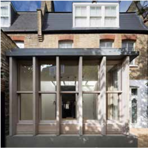
Right and above: extension to a house by Studio Carver, the elevation formed from timber fins with sash windows between
