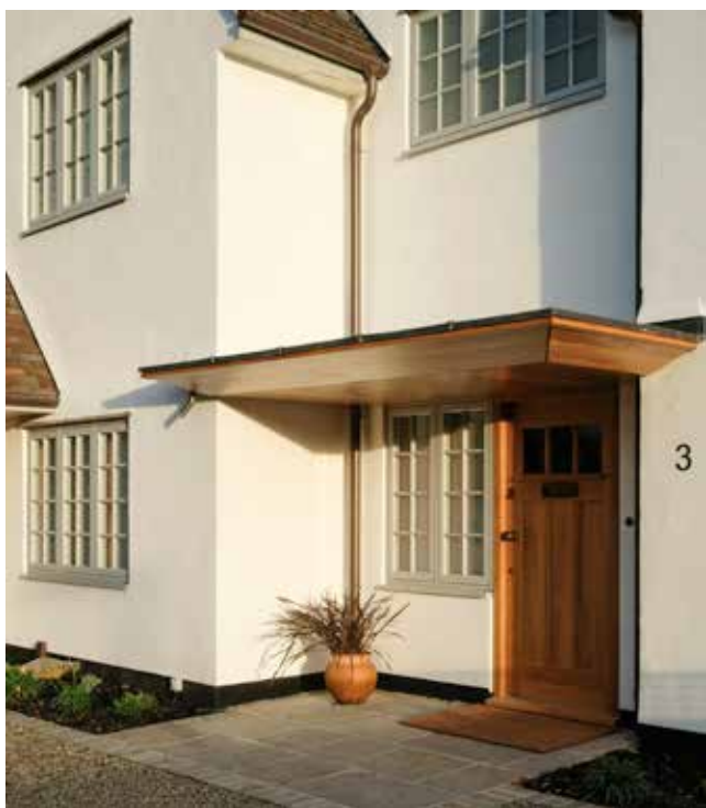
oak canopy and door with pigmented zinc rainwater goods at a recent project by NRAP in Cambridge's Storey's Way Conservation Area
