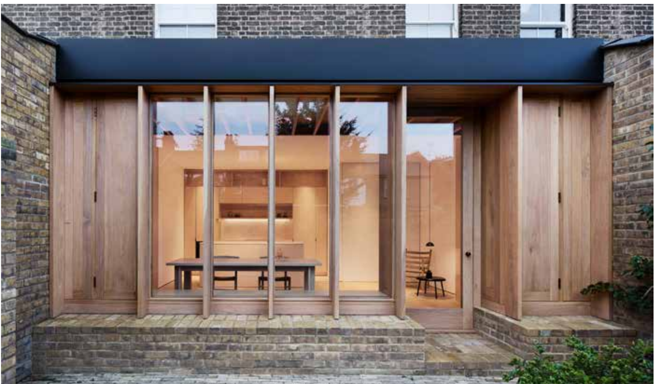
Right and below: extension to a house by O'Sullivan Skoufoglou, the elevation formed from timber fins with glazing or boarding between
