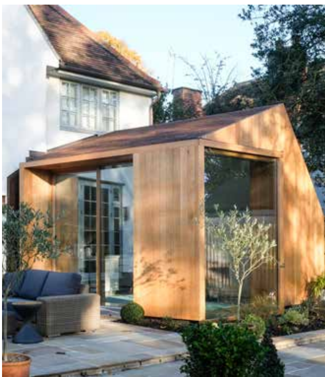
oiled oak boarding to an extension at a recent project by NRAP in Cambridge's Storey's Way Conservation Area
