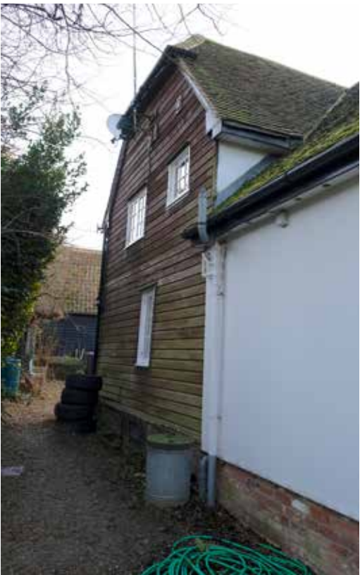
The east end of the house, which was clad with timber boarding in the early twentieth century
