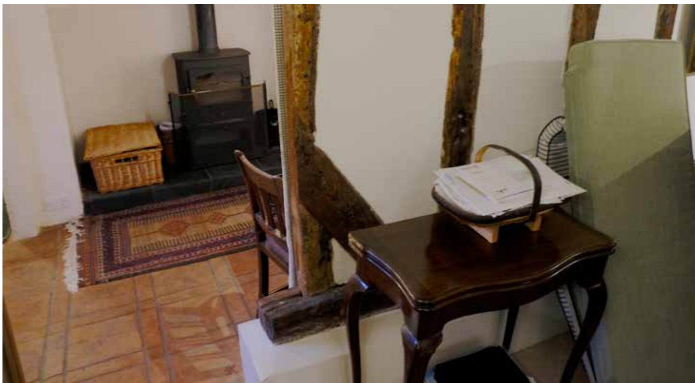
below: stub of the diagonal tie at the base of the wall between the present Kitchen and Dining Room suggesting that this wall was part of the original house and that the present opening was cut through the wall
