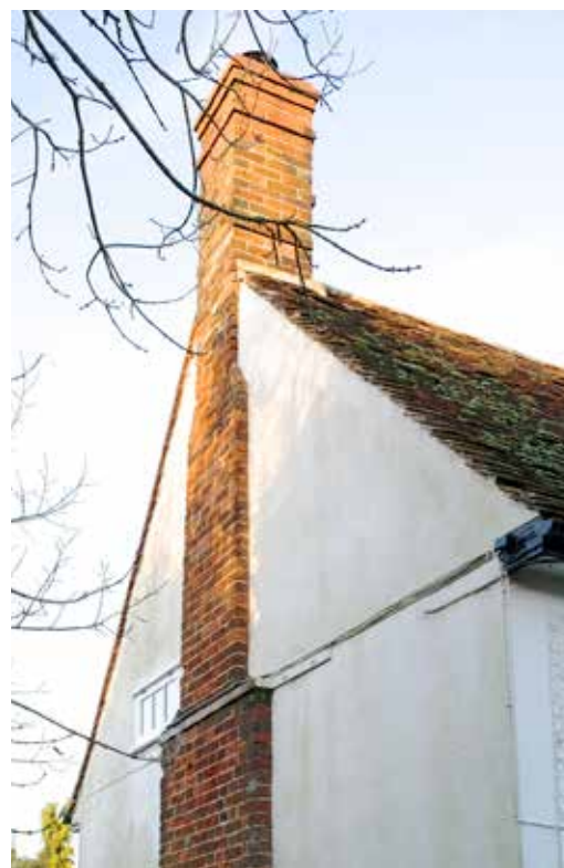
The nineteenth-century chimney on the west end of the house, the stack at the top has been rebuilt
