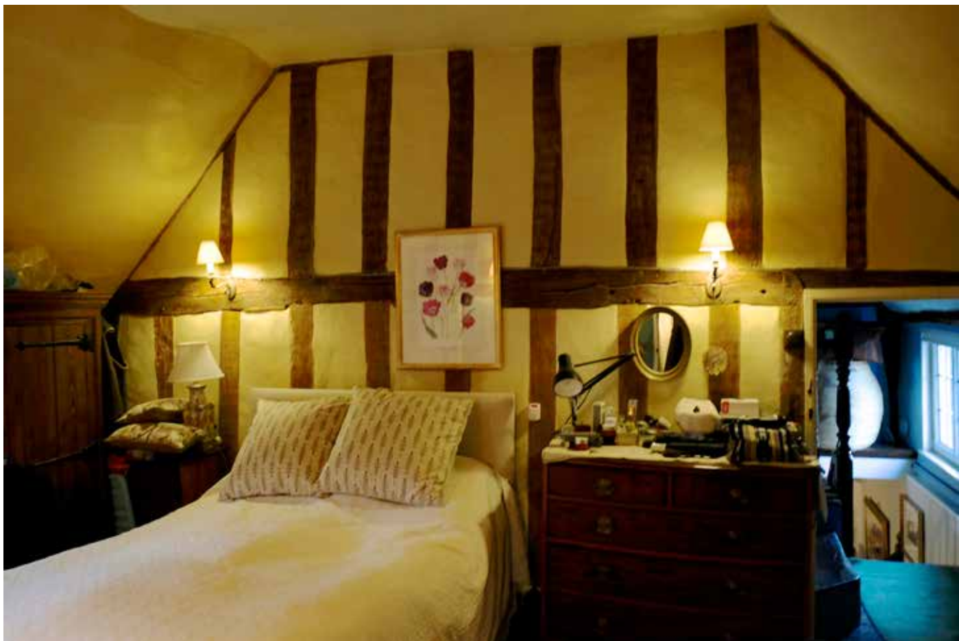
above: wall on the first floor marking the original western extent of the house with door cut through to nineteenth-century extension
