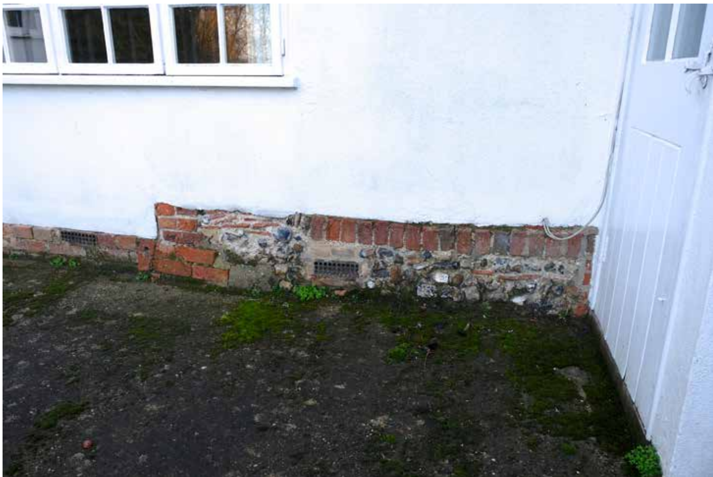
The masonry plinth to the north wall of the original house at the top of the terrace showing a mixture of flint, tile, old brick and modern brick
