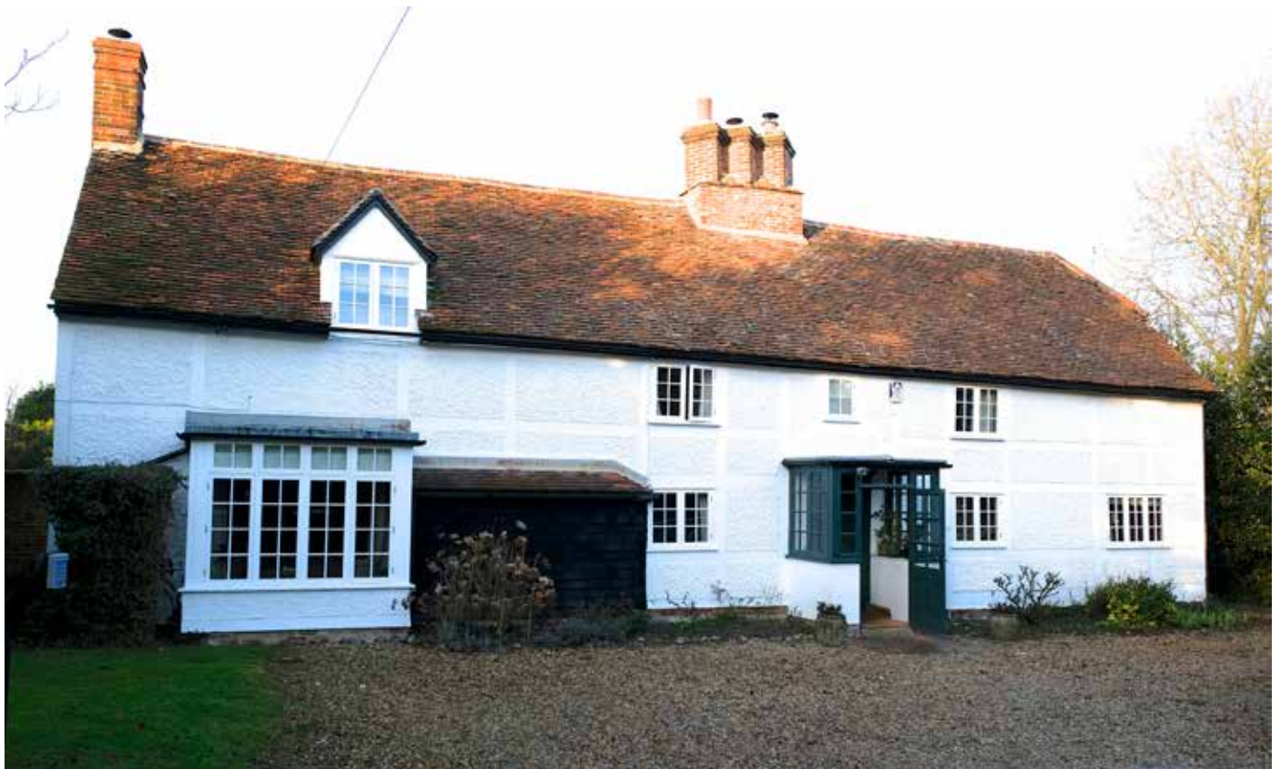
above: the south front of the house, the bay window and porch were added in the twentieth century
