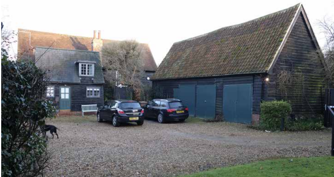
above: the space in front of the house with the Grade II-listed barn that sits on the southern site boundary to the right
