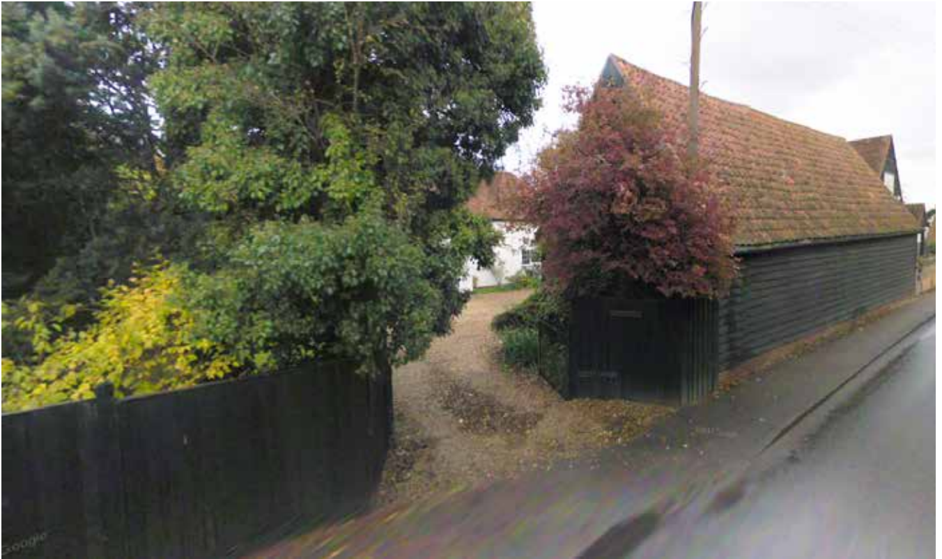
above: entrance to the site from Church End with the Old Granary barely visible beyond the boundary planting and the barn abutting the street, solid gates have been added to the drive opening since this photograph was taken
