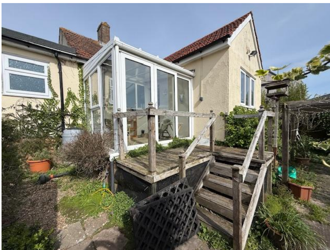
Figure 12: 5 Cambridge Road – Rear elevation, including conservatory
