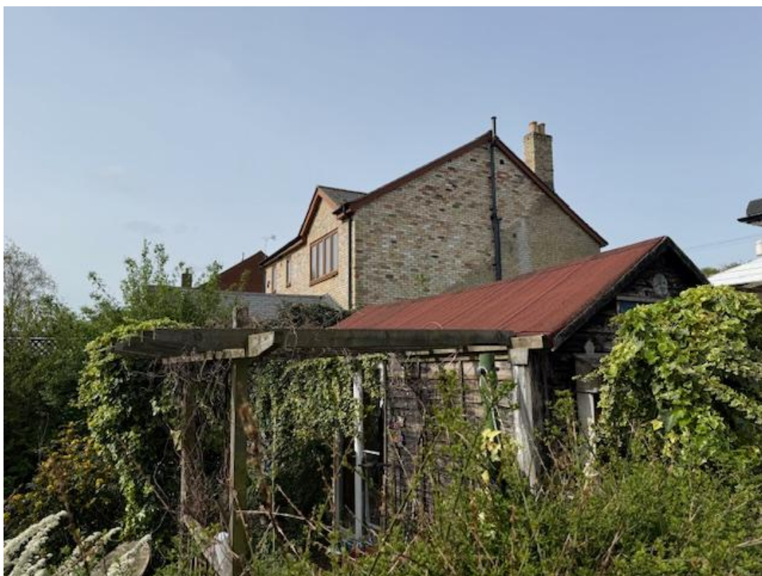
Figure 9: 5 Cambridge Road – Outbuilding & side elevation of 4 Cambridge Road
