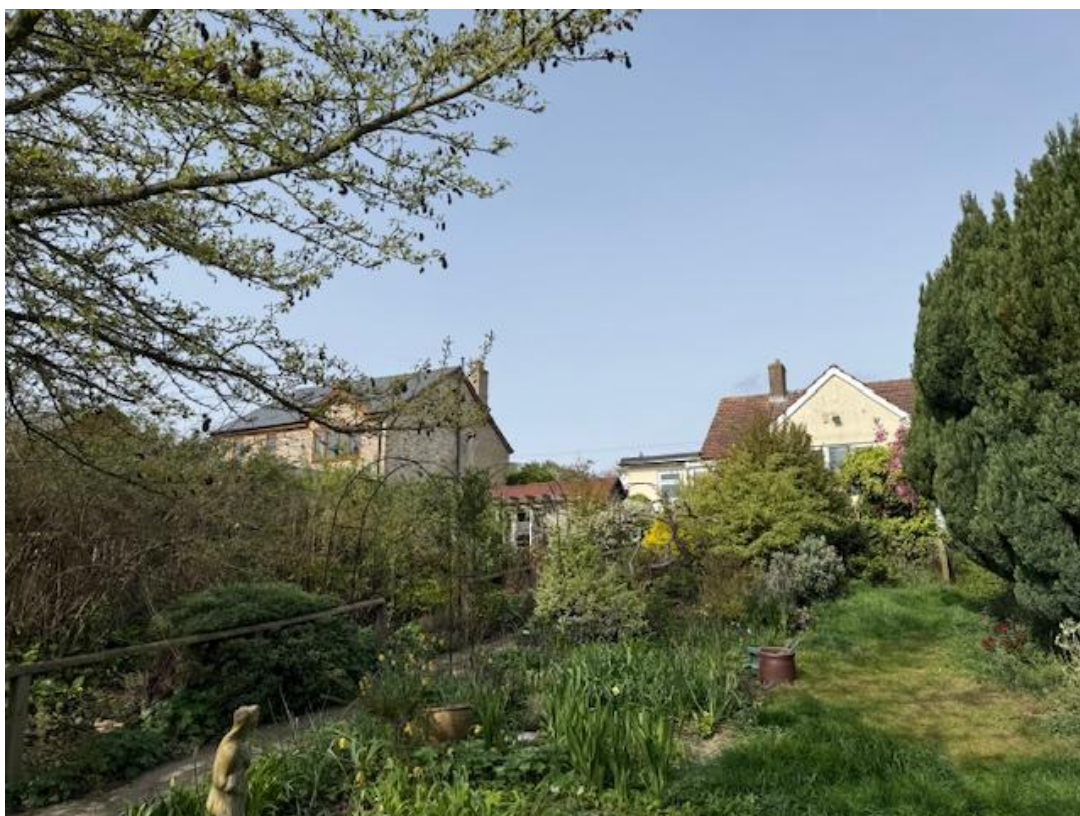
Figure 7: 5 Cambridge Road – Rear elevation & 4 Cambridge Road
