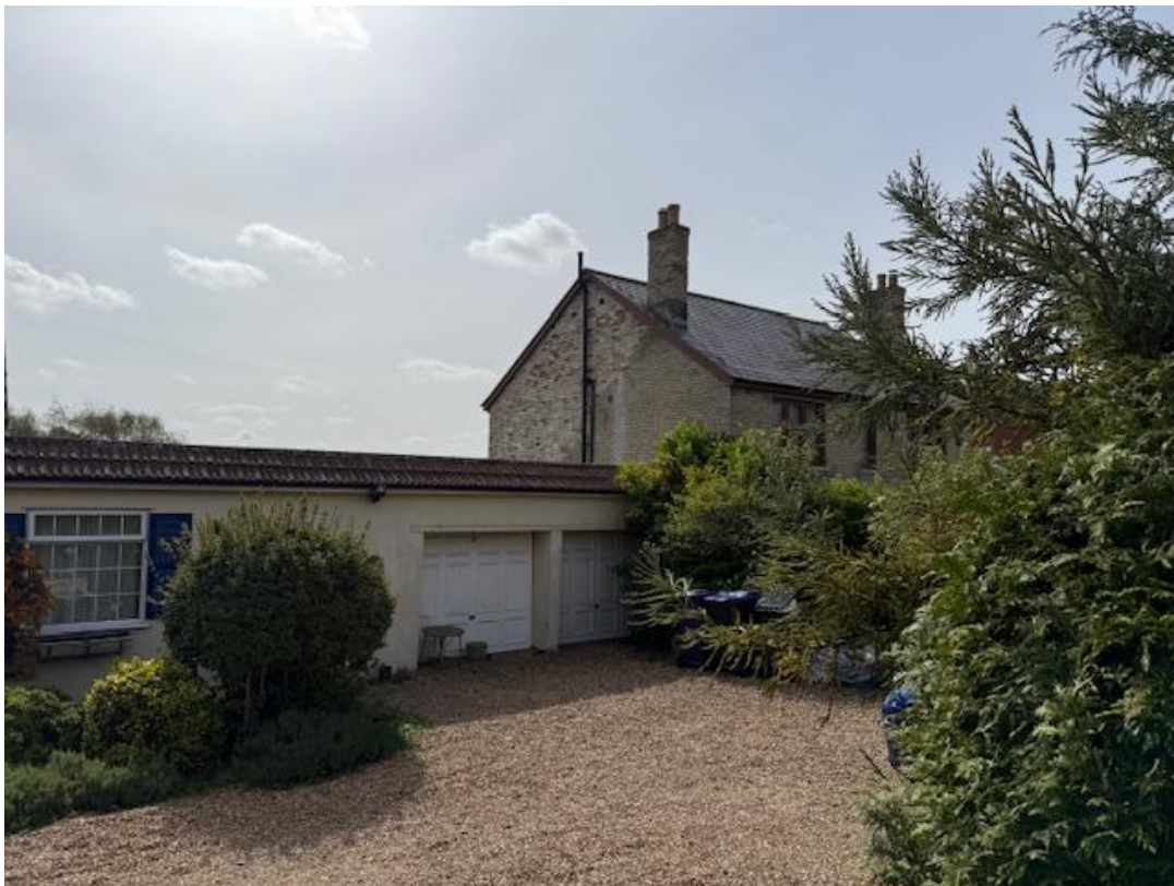
Figure 3: 5 Cambridge Road - Front Elevation & 4 Cambridge Road
