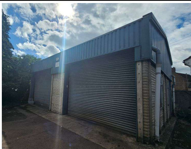
Photograph Eighteen: Workshop to southern corner of the site.
