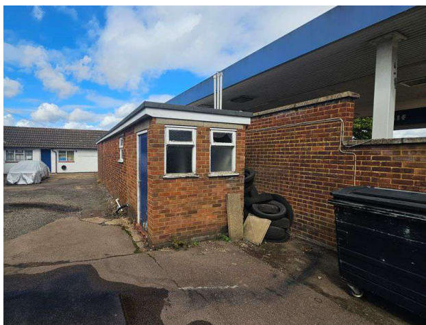
Photograph Sixteen: Toilet block to rear of forecourt sales building (with vents behind).
