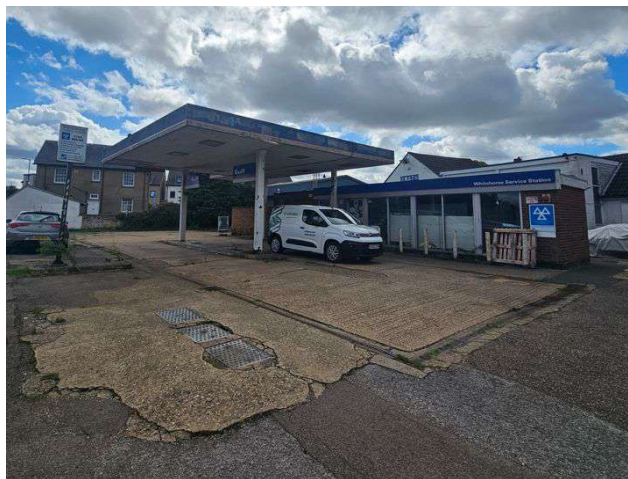
Photograph Four: Former forecourt area, showing sales building, canopy and forecourt interceptor (in foreground)
