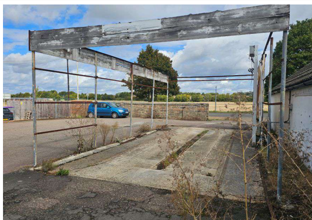
Photograph Twenty: Former car wash stand.
