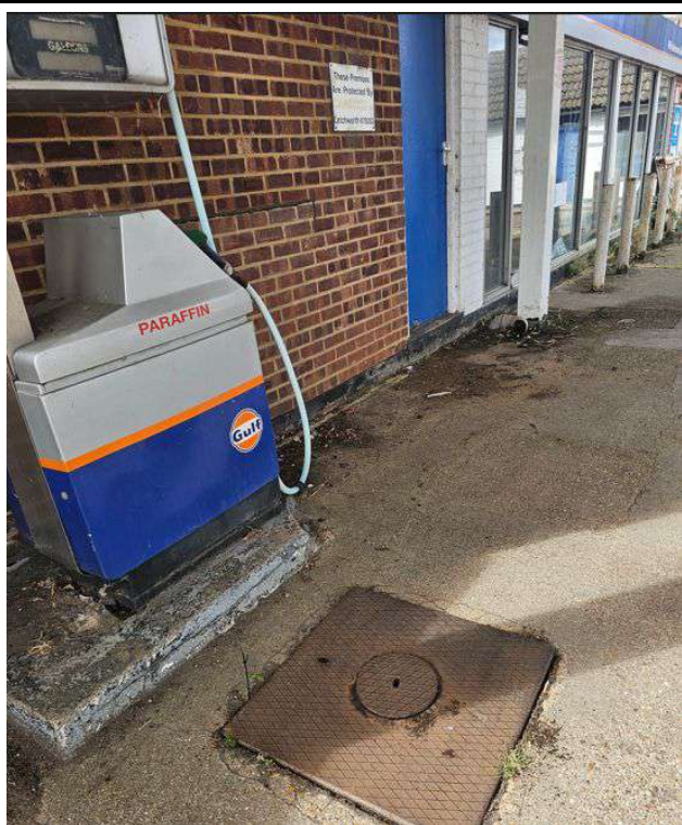
Photograph Six: Paraffin dispenser with adjacent tank access chamber
