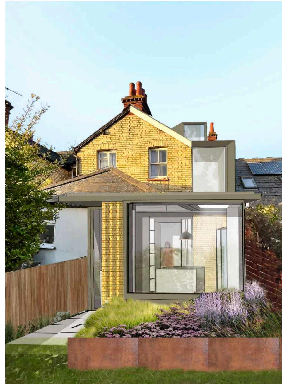
Chosen Iteration Combination of green tone aluminium cladding and decorative rainscreen buff brick cladding to match existing buff facing brick.
