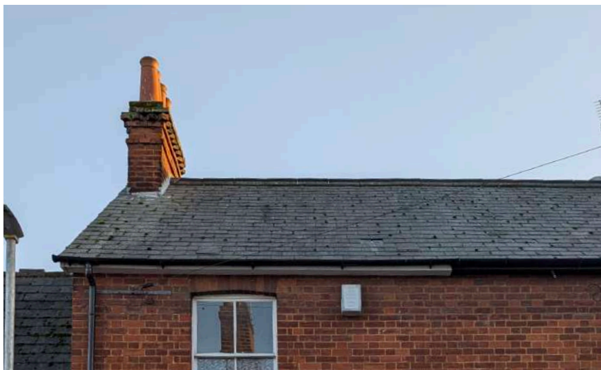
Existing slate tiled roof
