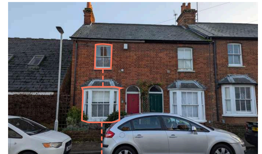
Existing timber frame windows of historic significance
