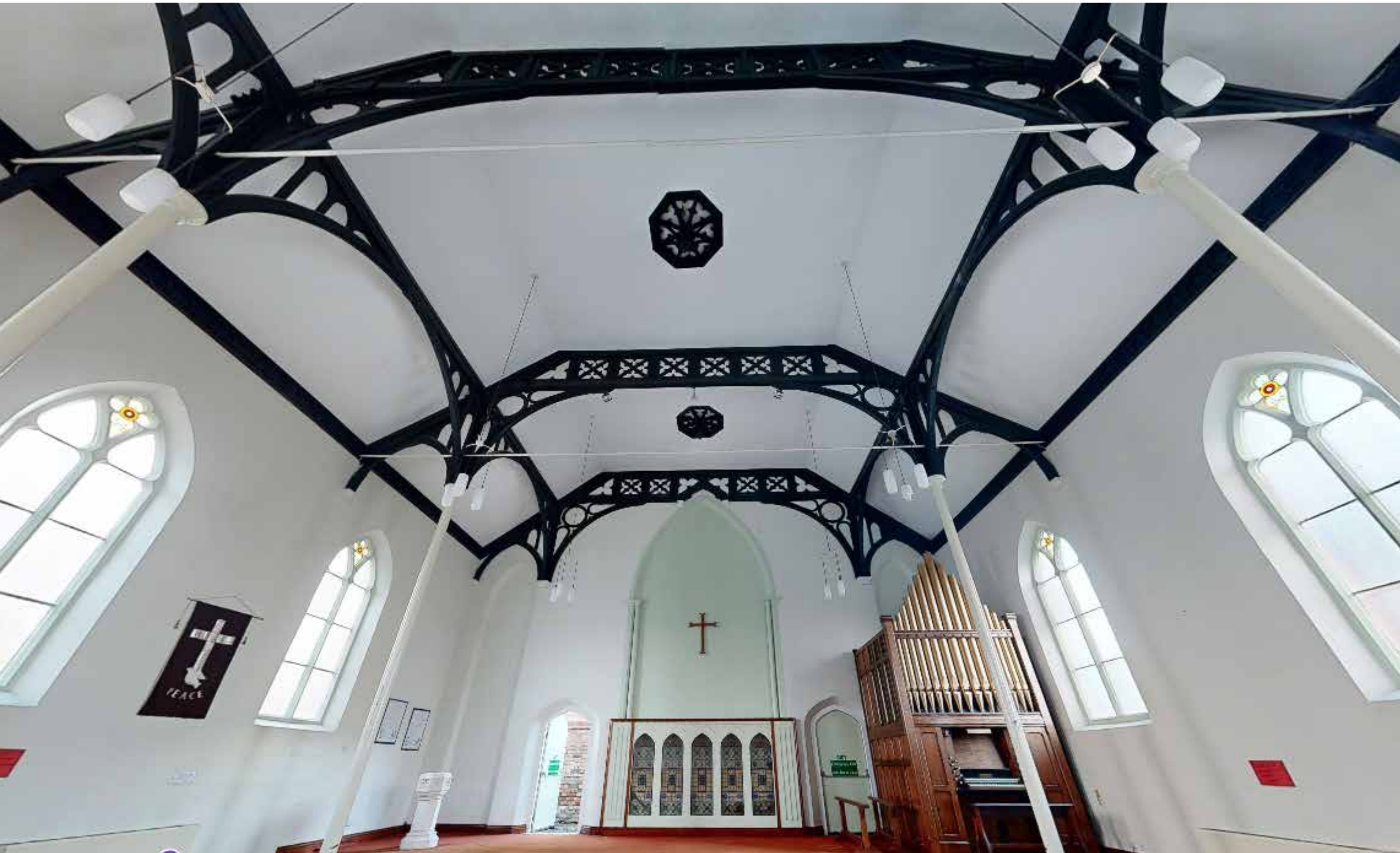
Fig. 07 : Internal view of the vaulted ceiling and original decorative features
