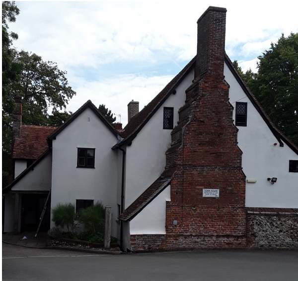
Photograph 5 – Existing Town House Side Elevation - windows to be replaced.
