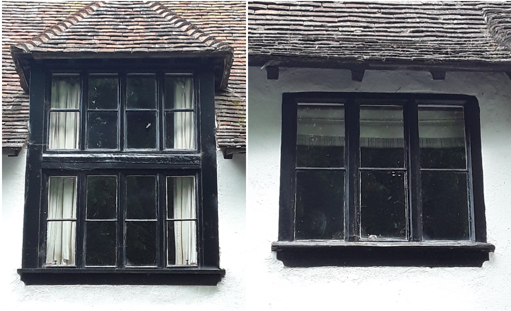
Photograph 2 – Existing Town House first floor windows to be replaced adjacent to Church End.
