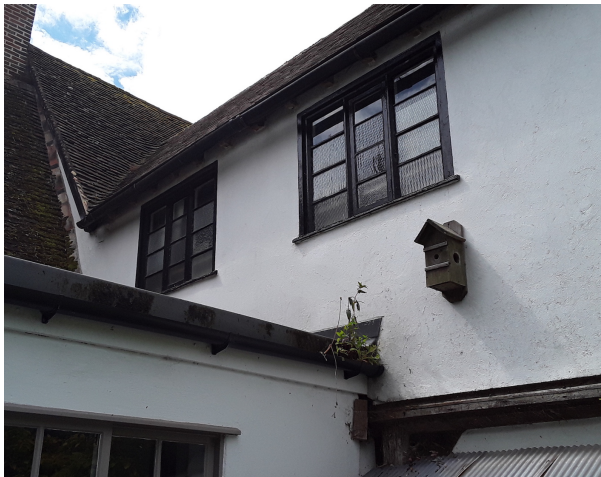
Photograph 4 – Existing Town House Kitchen first floor windows to be replaced.
