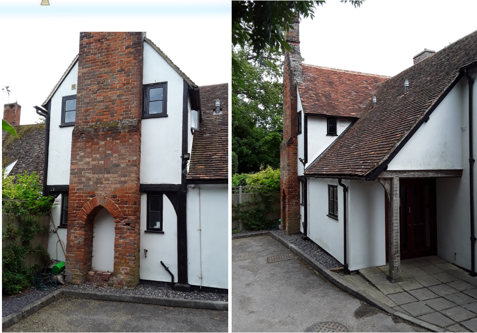
Photograph 3 – Existing Town House Kitchen first floor windows to be replaced.
