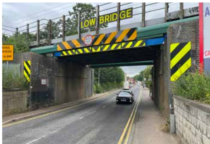
▲ Railway bridge over A507 North Road/Station Road
