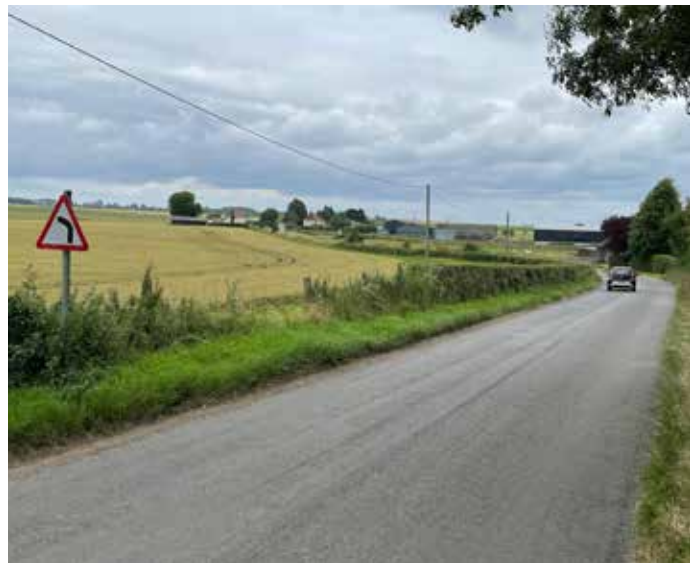
▲ Top: Landscape north of the railway line Bottom: Western end of Bygrave Road looking east
