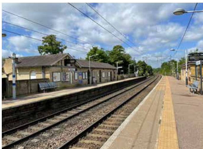
▲ Baldock Railway Station
